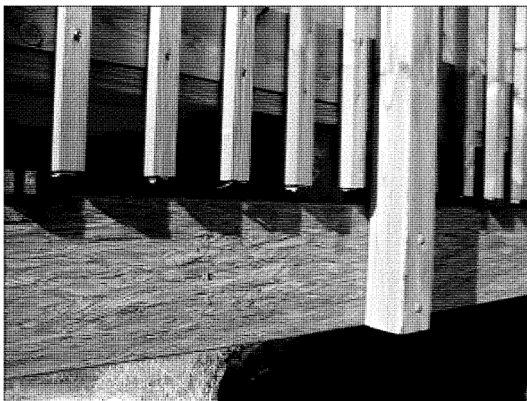
Figure 13. Pressure-treated parallel strand lumber (PSL) beams were used as supports for this trail bridge.
