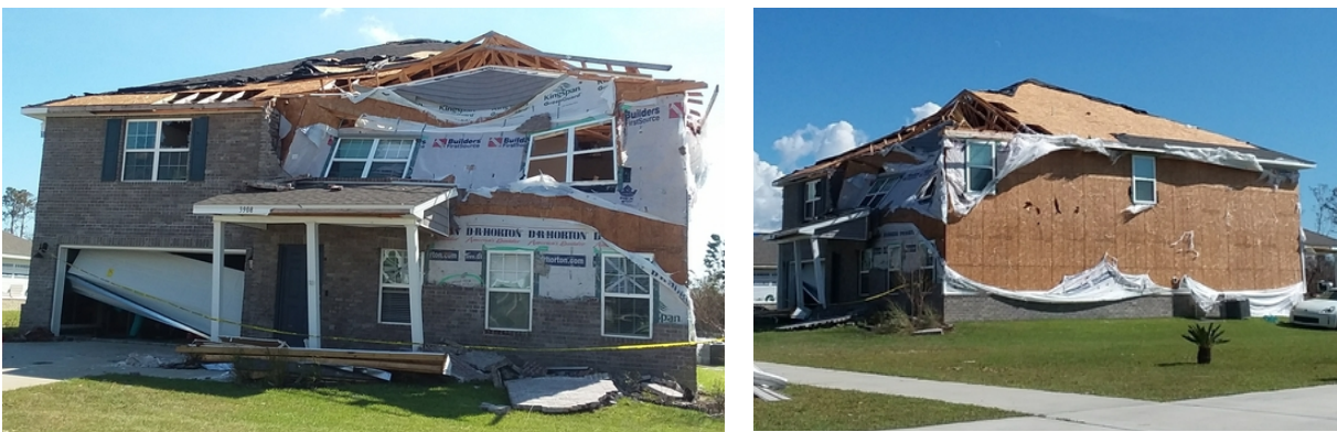
Figure 22. Damage to a 2016 home in the Magnolia Hills subdivision in Panama City, FL. The estimated peak gust wind speed here was 57 m/s, with an ASCE 7-10 design wind speed of 59 m/s.
