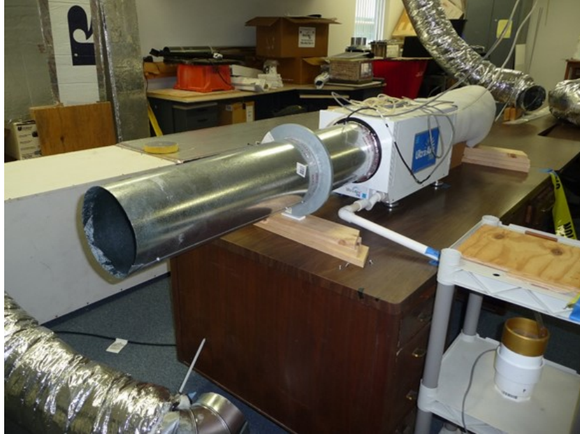
Figure 4. Dehumidifier shown with return air flow station and condensate drain to tipping bucket on a stand.
