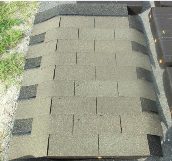
Figure 31: Membrane installed on all edges to prevent uncontrolled moisture travel
