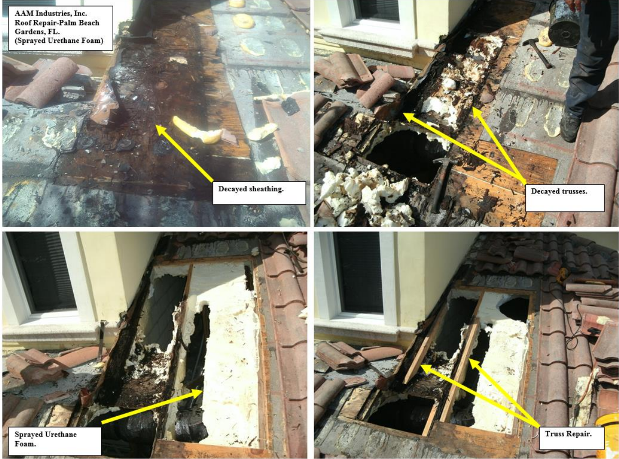
Figure 8: Moisture damage around a gable dormer to an unvented attic with ccSPF.
