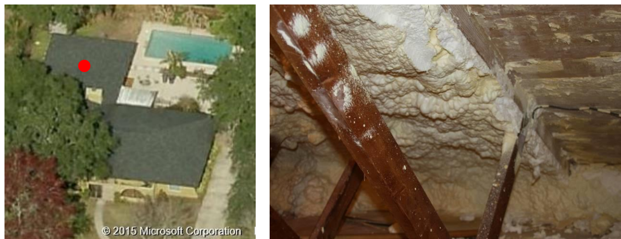
Figure 12: (Left) Aerial view of Home 2. The red dot indicates the approximate location of the photo to the right. (Right) ocSPF installed in the attic space. The truss shown is directly over the garage wall. SPF to the right of the truss, over the garage, has been removed by the homeowner.
