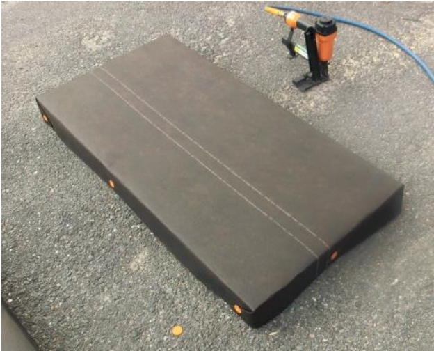
Figure 31: Membrane installed on all edges to prevent uncontrolled moisture travel
