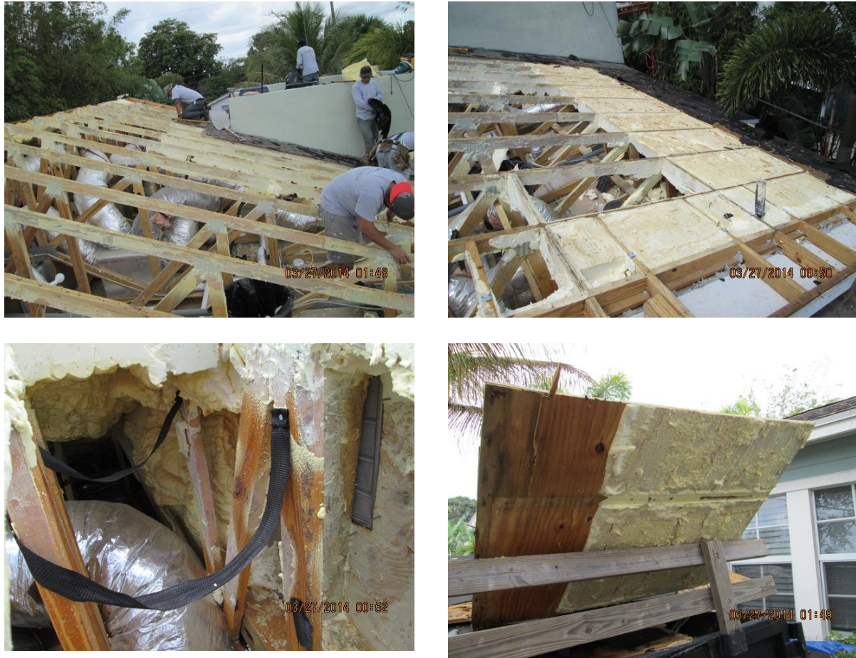
Figure 9: Evidence of moisture buildup in home installed with ccSPF. Note the moisture on both the sheathing and wood framing
