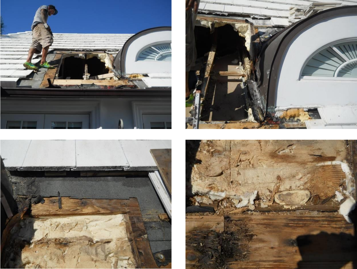
Figure 7: Moisture damage in an unvented attic with ccSPF. Moisture was particularly event around the visible dormer (Courtesy of Mark Zehnal).
