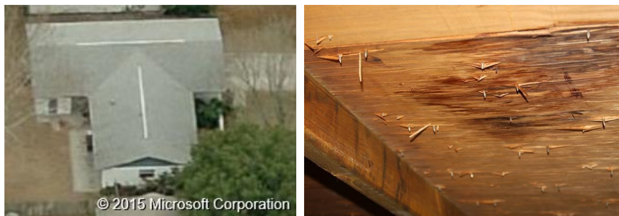
Figure 13: (Left) Aerial view of Home 3; (Right) Apparent water damage in the plywood sheathing. No moisture was present at the time of inspection, and no evidence of past moisture was evident in the insulation below.
