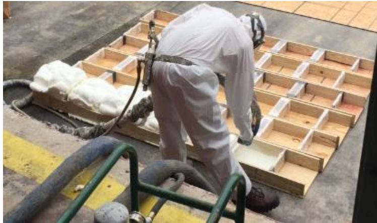
Figure 18: Installation of open-celled SPF insulation
