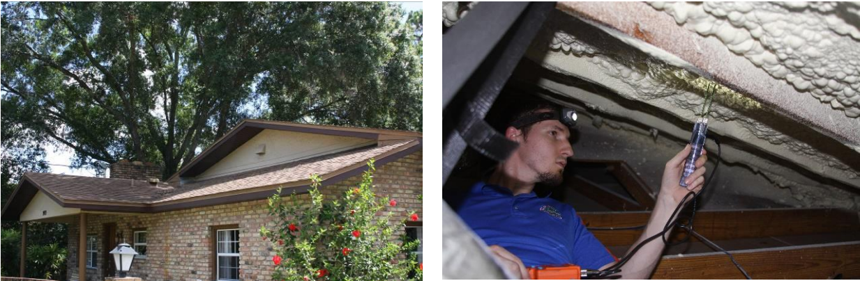
Figure 11: (Left) View of the front of the house from ground. (Right) View from inside the attic showing the ccSPF and a moisture content measurement being taken.
