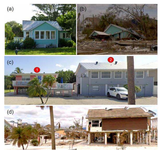
Importance of freeboard elevation to survivability, including (a) before and (b) after views of a singlefamily home on Estero Island constructed in 1950 that collapsed during Hurricane Ian; (c) before and (d) after views of two homes with disparate performance on Estero Island. Home (1) was constructed in 1956, while home (2) was constructed in 1950, but home (2) was elevated approximately 3 ft higher than home (1) and its breakaway walls performed as intended. 7
