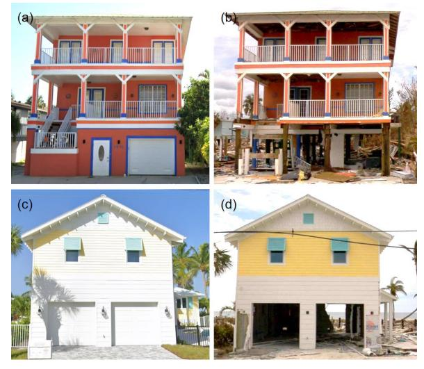
Examples of the performance of breakaway walls during Hurricane Ian, including (a) before and (b) after views of a home on Estero Island constructed in 2000 with acceptable performance of the breakaway walls; and (c) before and (d) after views of a two-story structure with garage at ground level constructed in 2020 in which the breakaway CMU walls on the back side of the structure only partially broke away.
