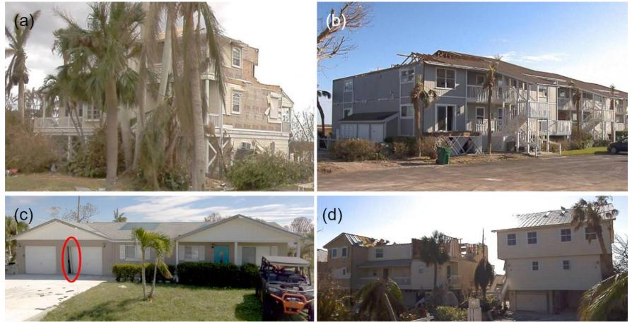
Examples of poor wind performance on the barrier islands, including (a) a 3-story home constructed in 1999 with partial roof structure removal and wall collapse in the top story, (b) gable end roof structure loss in apartment buildings constructed in 1986; (c) garage door framing blown inward in a home constructed in 1967; (d) roof structure failure in one home adjacent to loss of metal roof cover in another, both of which were constructed in 1978.
