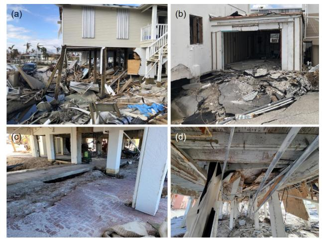
Examples of scour, uplift, and other surge effects on buildings during Hurricane Ian, including (a) debris transport and breakaway wall performance, (b) scouring and pavement washout, (c) scour around piers, and (d) effects of hydrodynamic uplift forces on a woodframed floor system
