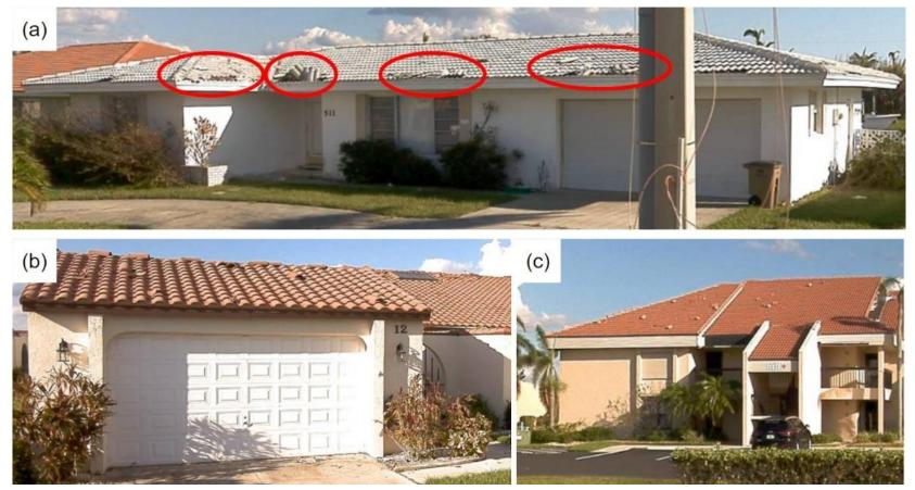
Illustrative examples of damage to tiled roofs, including (a) tile uplift (indicated by red ellipses) concentrated along the eaves of a single-family home in Punta Gorda constructed in 1969; (b) loose tiles in the field and ridge regions of the roof on a condominium in Punta Gorda, FL constructed in 1989; and (c) isolated loose tiles on a roof on a multi-family residential unit also in Punta Gorda, FL constructed in 1990.
