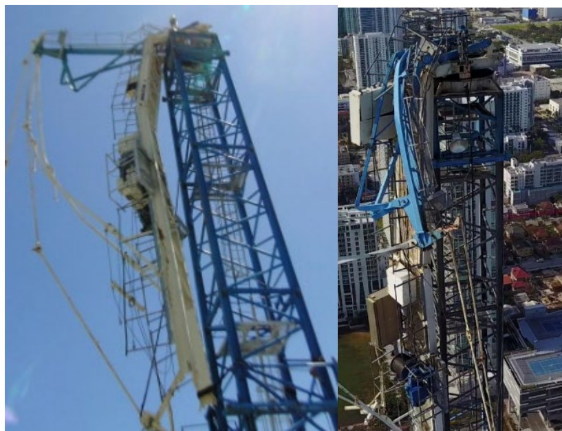
Figure 5-7. One example of the failed cranes in South Florida during Hurricane Irma. [21]
