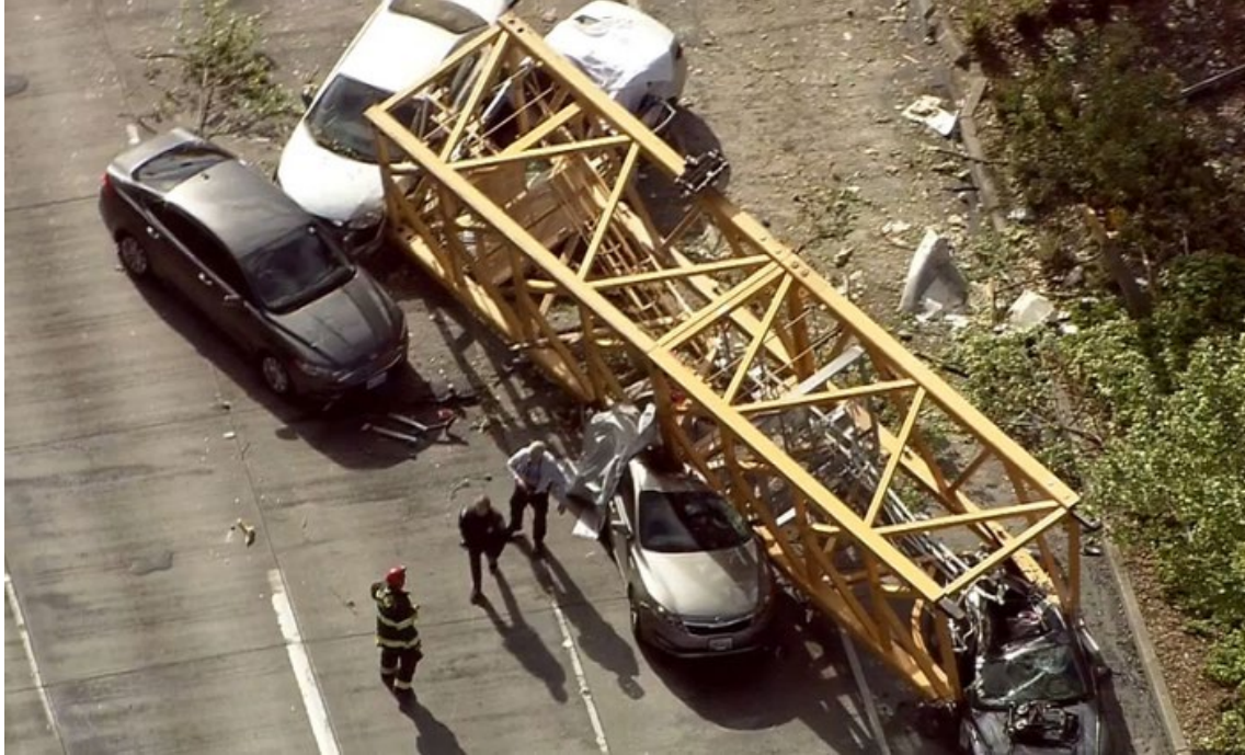
Figure 5-11. Crane failure in Seattle, Washington. (KIRO7.com)
