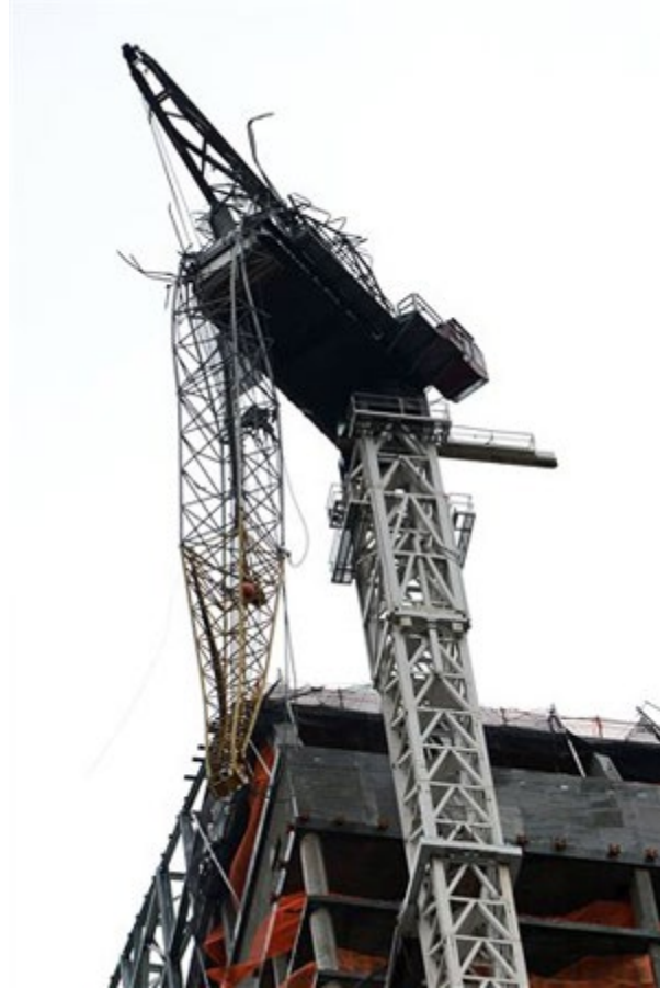
Figure 5-5. Tower crane destroyed during Hurricane Sandy in New York City. [20]
