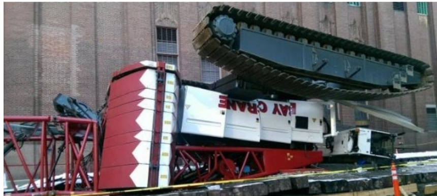
Figure 5-3. Overturned crawler crane in New York City. [16]
