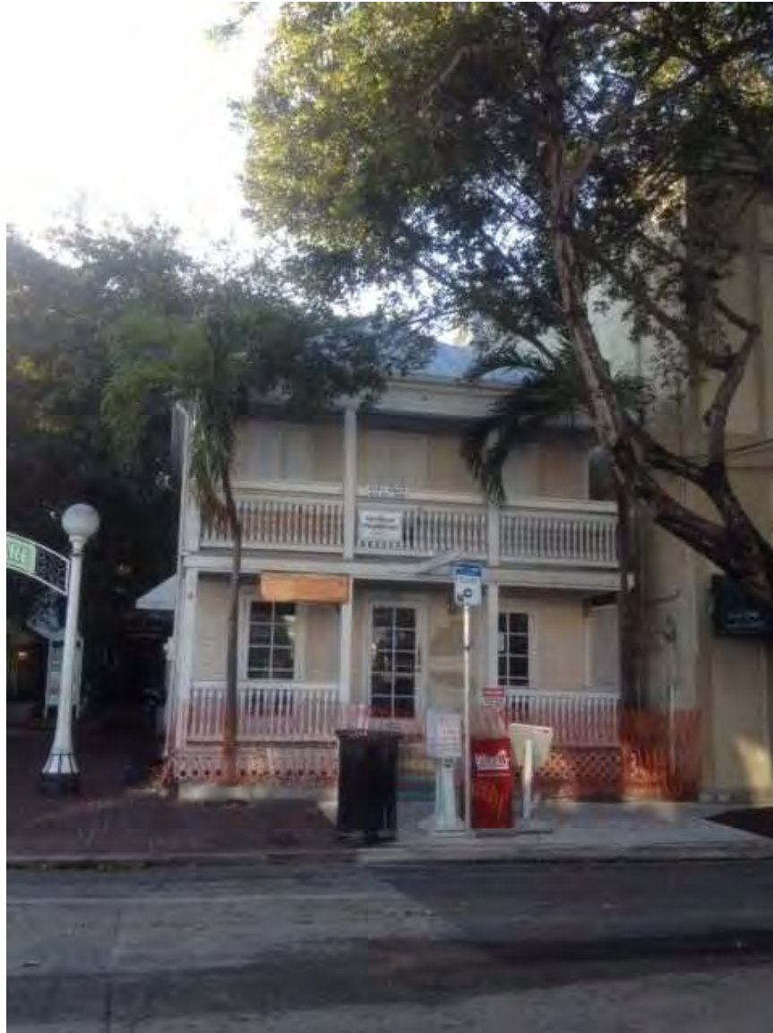
506 Southard Street main façade.
