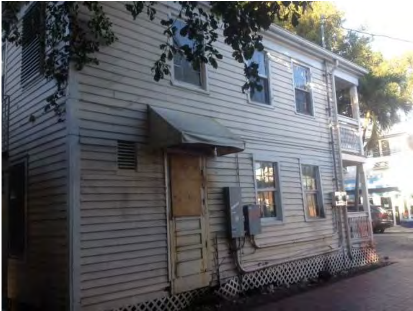
506 Southard Street east façade.
