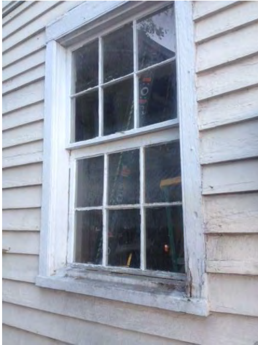
506 Southard Street one of the original windows.
