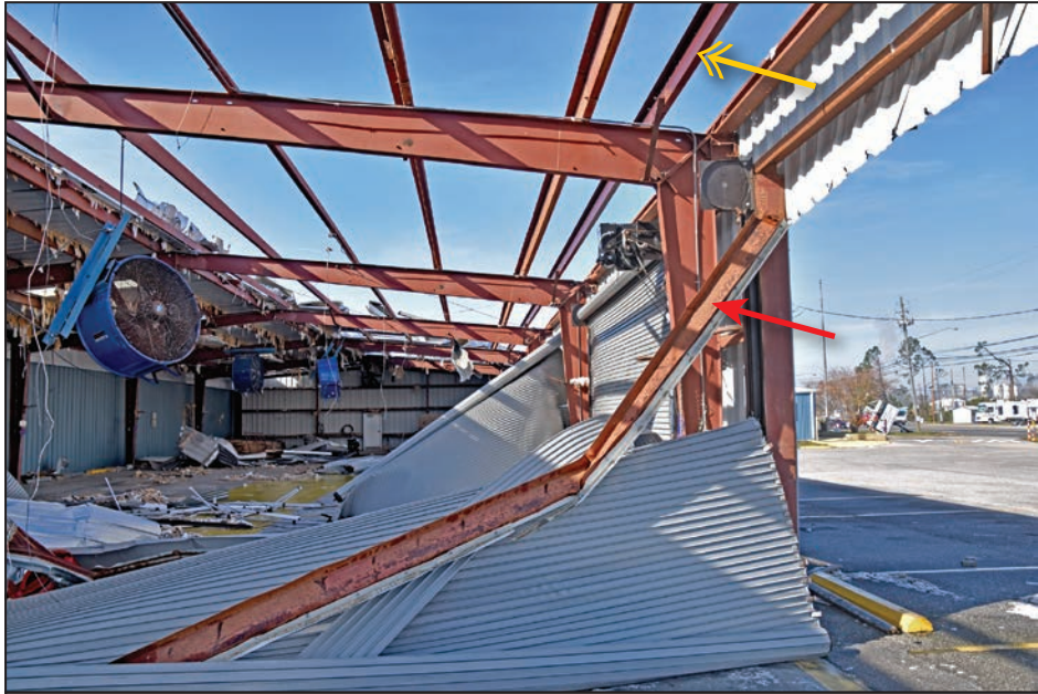
Figure 8: View of the new purlin
