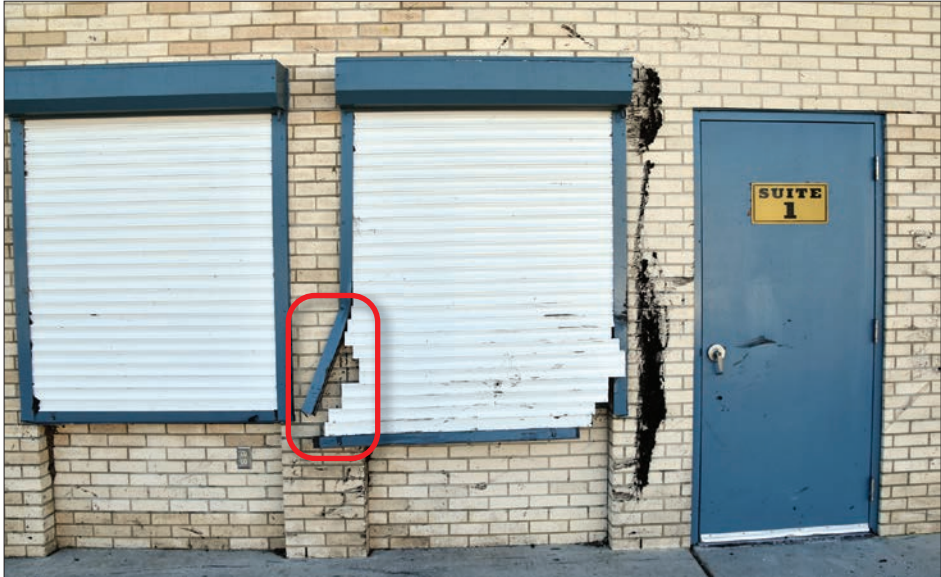
Figure 3: These shutters were struck by wind-borne roof membrane debris; distorted jamb and sill frame indicated by red rectangle
