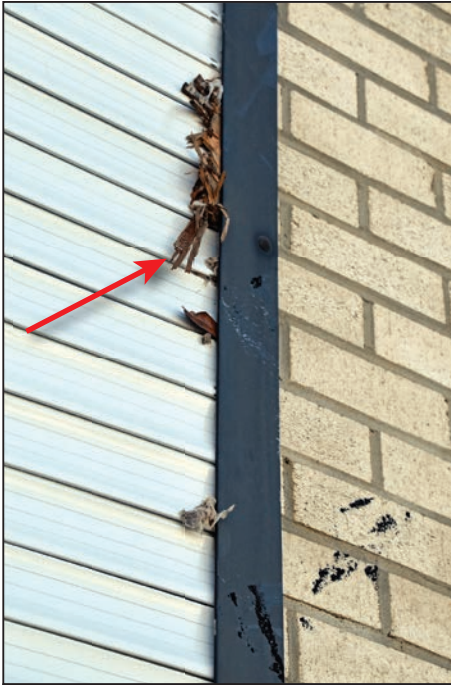
Figure 3: These shutters were struck by wind-borne roof membrane debris; distorted jamb and sill frame indicated by red rectangle
