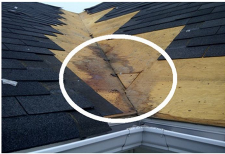
Result of an improperly flashed valley!!!
