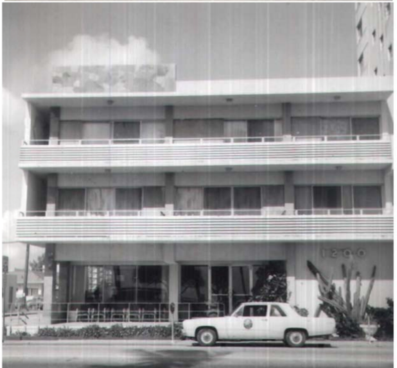
TOP PHOTO: 1959 EAST AND SOUTH ELEVATIONS SHOWS ORIGINAL FULL HEIGHT WINDOWS AT FRONT CORNER LOBBY AREA ON FIRST FLOOR. (9)
