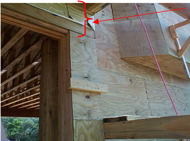
Photo C.2 shows: Exterior view of sheathing as described above.
