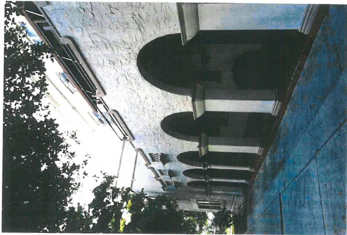
Front loggia note: Block columns
