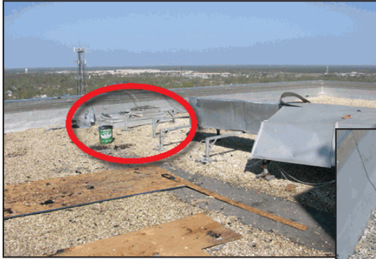
Figure 5. Two large openings remained (circled area and inset to the right) after the ductwork on this roof blew away.
