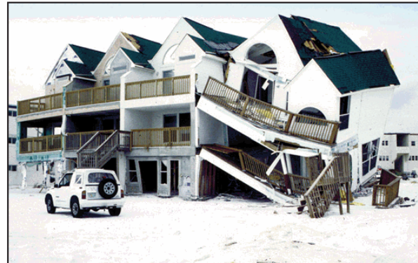
Figure 1. Failure of wood-frame walls used to support a coastal building, which was subjected to shallow flooding, small waves, and floating debris (Hurricane Opal).
