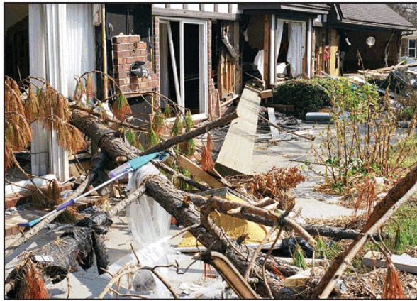
Figure 5. Damage to light frame walls due to floating debris and small waves. The damaged home was in the third row back from a bay shoreline (Hurricane Ivan).
