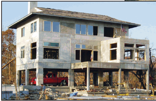
Figure 13. Pass Christian, Mississippi, home elevated on reinforced concrete columns in Zone A, with the bottom of the floor beam elevated approximately 9 feet above the BFE. Although Katrina flooding was approximately 4 feet above the top of the lowest elevated floor, the home sustained no structural damage. All other buildings in the vicinity were destroyed.
