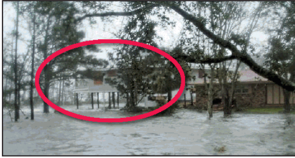
Figure 13. Pass Christian, Mississippi, home elevated on reinforced concrete columns in Zone A, with the bottom of the floor beam elevated approximately 9 feet above the BFE. Although Katrina flooding was approximately 4 feet above the top of the lowest elevated floor, the home sustained no structural damage. All other buildings in the vicinity were destroyed.
