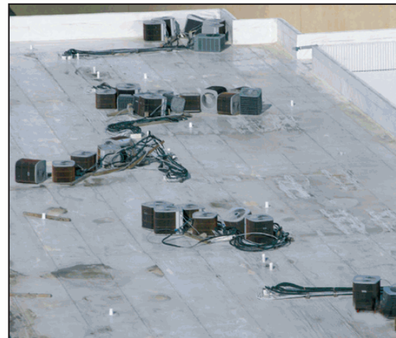
Figure 6. Sleeper-mounted condensers displaced by high winds.
