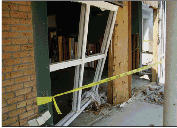
Figure 3. Failure of wood-frame wall, brick veneer, and windows as a result of 4 feet of stillwater flooding and small waves (Hurricane Katrina).
