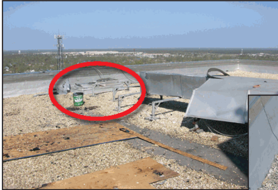
Figure 5. Two large openings remained (circled area and inset to the right) after the ductwork on this roof blew away.
