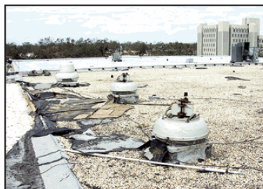
Figure 3. Cowlings blew off two of the three fans shown in this photo. Cowlings can tear roof membranes and break glazing.
