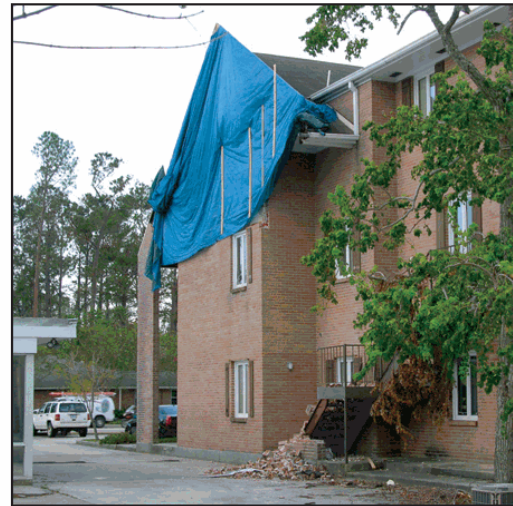
Figure 2. The upper portion of the brick veneer at this apartment building collapsed. Pedestrian and vehicular traffic in the vicinity of the damaged wall were vulnerable to injury and damage if remaining portions of the wall were to collapse during subsequent storms.
