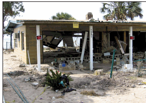
Figure 2. Masonry walls destroyed by 3 feet of stillwater flooding and small waves (Hurricane Dennis).
