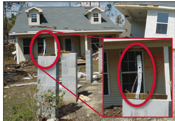
Figure 8. Post-Katrina investigations showed that many buildings were attached to foundation piers with light gauge metal straps. These straps failed in many instances. A stronger (preferably bolted) connection is recommended when attaching Coastal A Zone buildings to their foundations.
