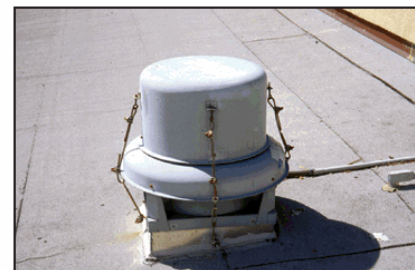
Figure 4. To overcome blow-off of the fan cowling, this cowling was attached to the curb with cables.
