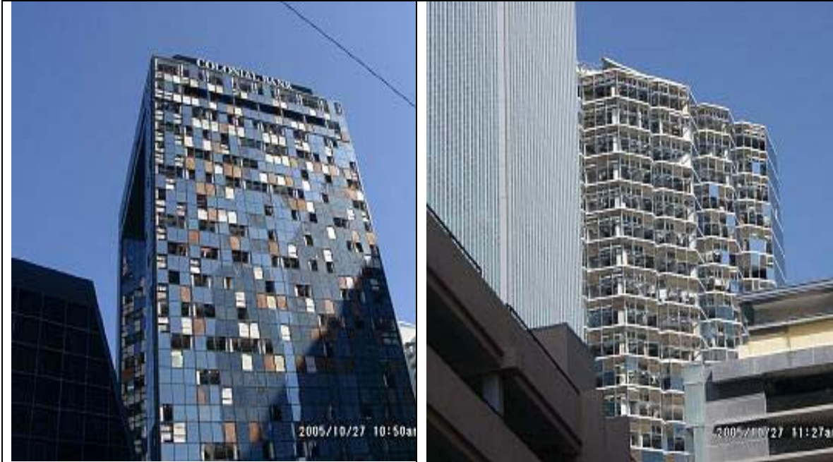
Some older apartment buildings in downtown Miami, near the scene of major destruction fared very well, with only minimal damage to patio glass panels.
