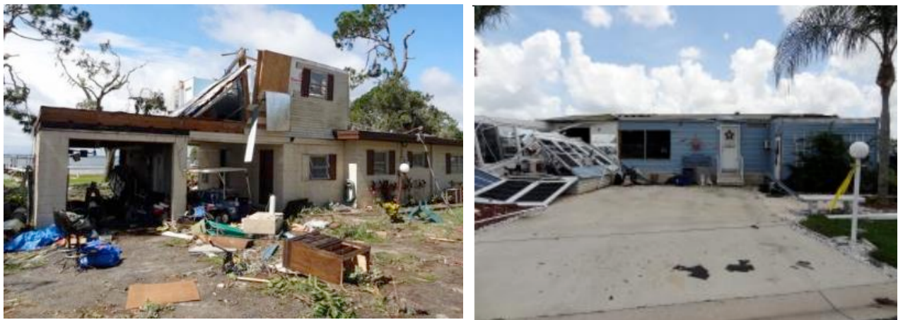
Figure 12: Post-2012 Lake Placid (Highland County) tornado damage showing EF2 damage (left) Post-2012 Vero Beach (Indian River County) tornado damage showing EF1 damage (right)
