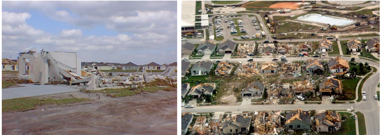
Figure 11: (Left) A destroyed concrete block and stucco home in Kissimmee, FL during 1998 F3 tornado ( http://www.srh.noaa.gov/mlb/?n=kissimmeepics ), (Right) Damaged homes in Lakeside subdivision in Kissimmee, Florida. The 1998 F3 tornado moved from the upper right to the lower left, narrowly missing a school. ( http://www.nws.noaa.gov/os/assessments/pdfs/cntrfl.pdf )
