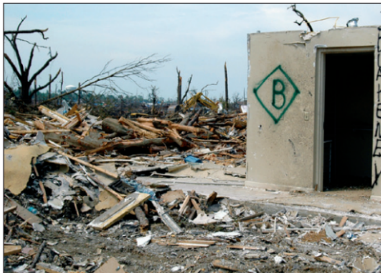
Figure 16: A hardened room in a residence Tuscaloosa, AL whose door failed in the April 27, 2011 tornado (source: FEMA (2012))
