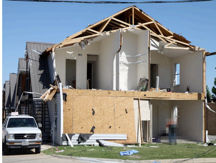
Figure 21: Wall connection failures from tornado damage
