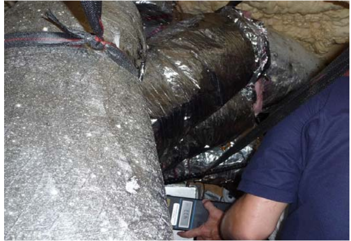
Testing the ERV's airflow.
