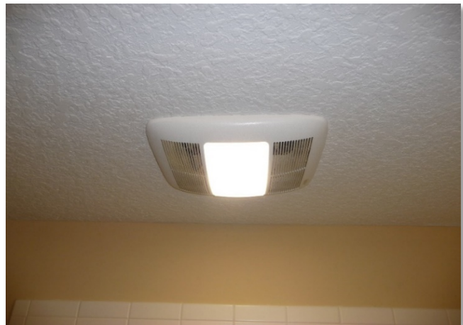
Figure 3. 3-way switchable master bath fan with light.
