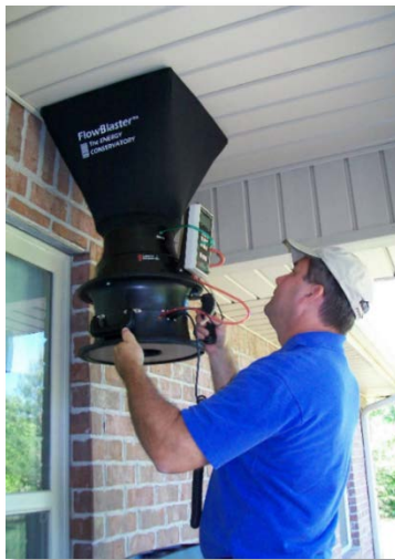
Figure 1. Measuring outdoor air flow of a runtime ventilation system using a FlowBlaster.
