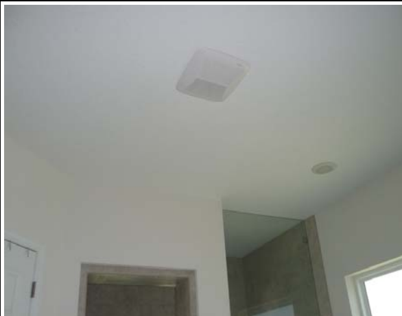
Bathroom exhaust fan.
