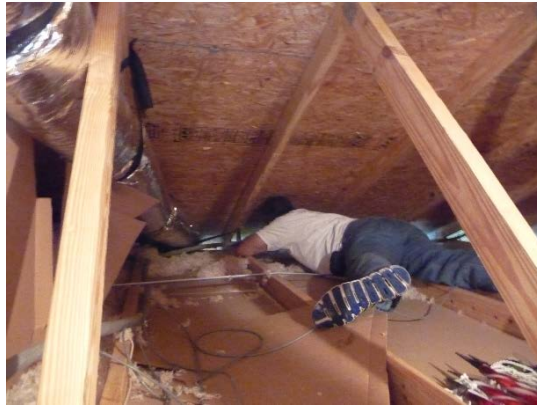
Figure 4. Measuring clearance for outdoor air duct at exterior wall / roof junction.
