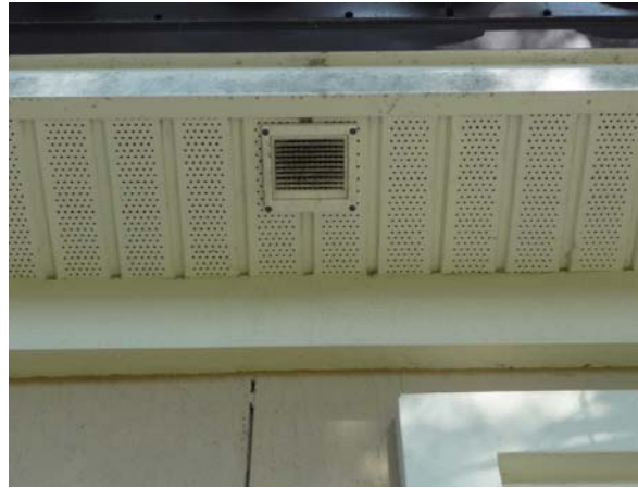
Bath exhaust grille in soffit.
