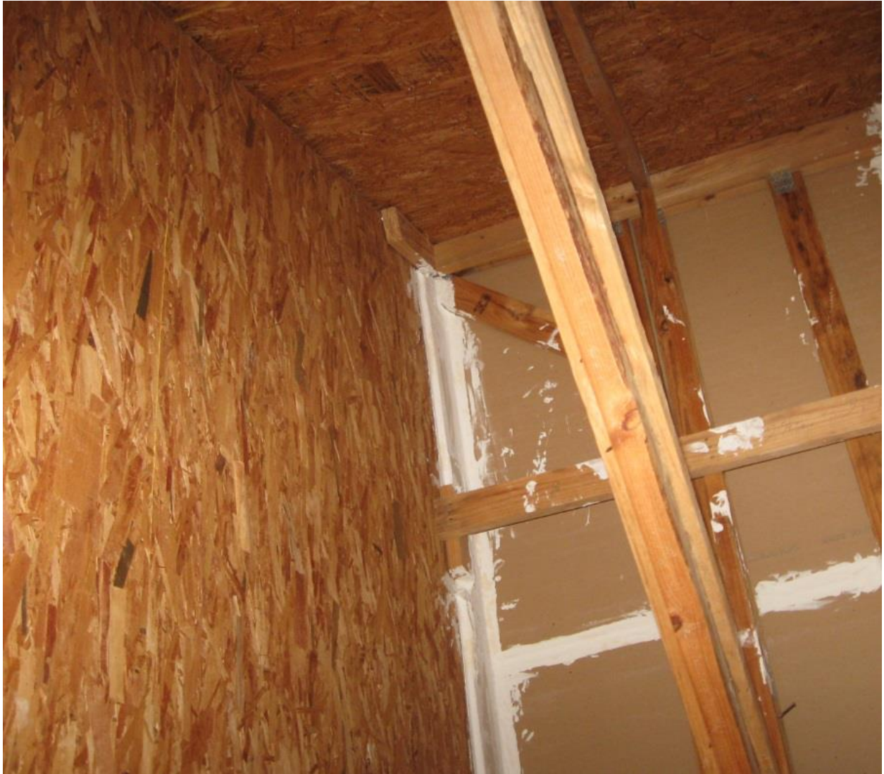
Picture 04 – Draftstopping with both Plywood and Gypsum
