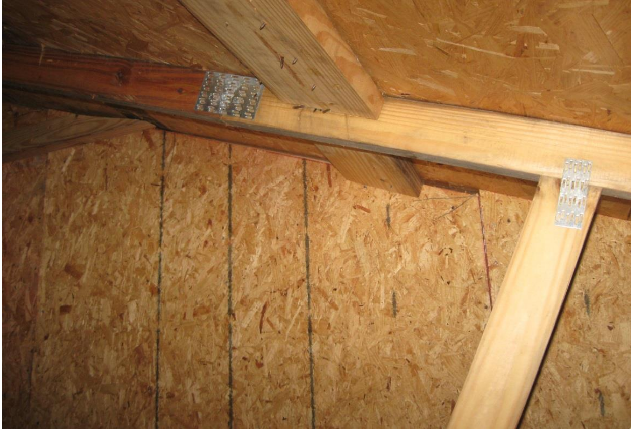
Picture 01 – Typical Plywood Draftstopping
