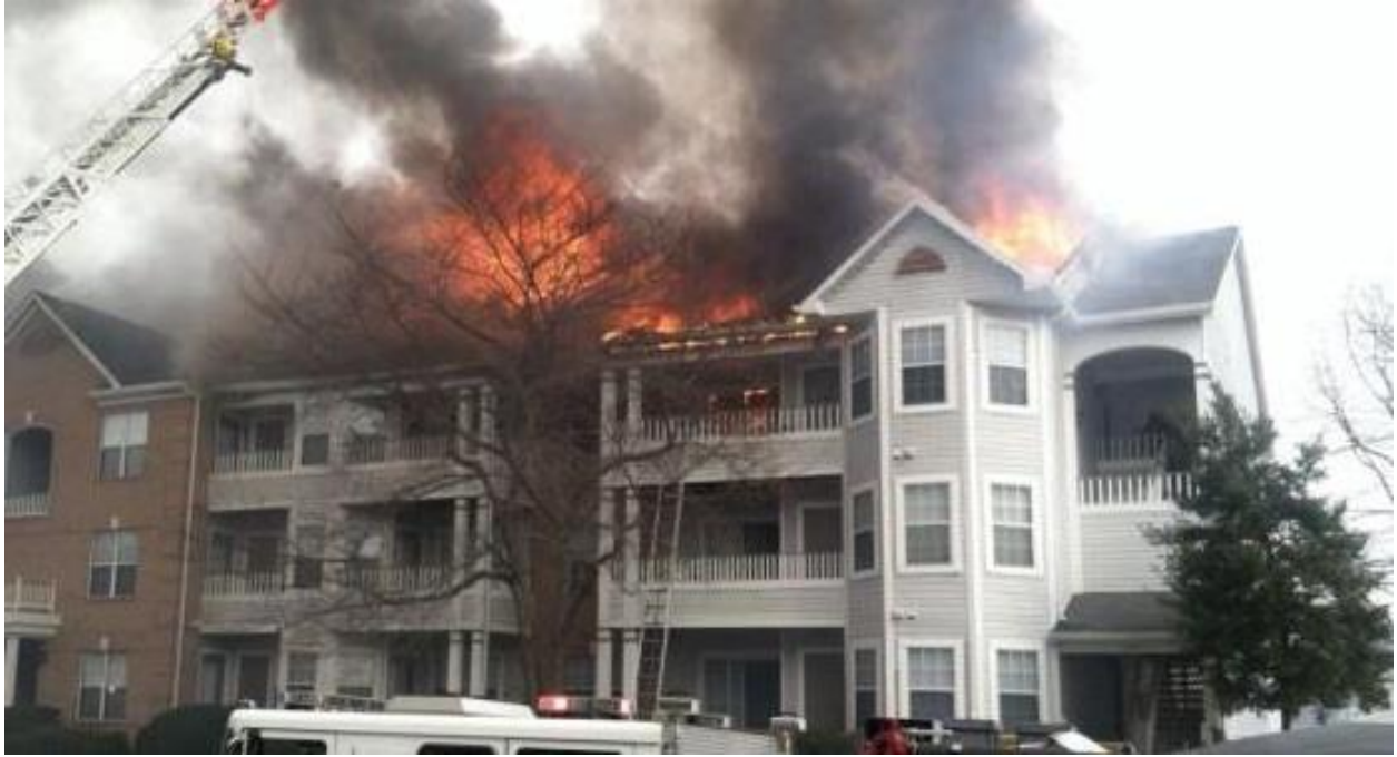
Picture 19 – Lightning Strike in Wood Attic.
