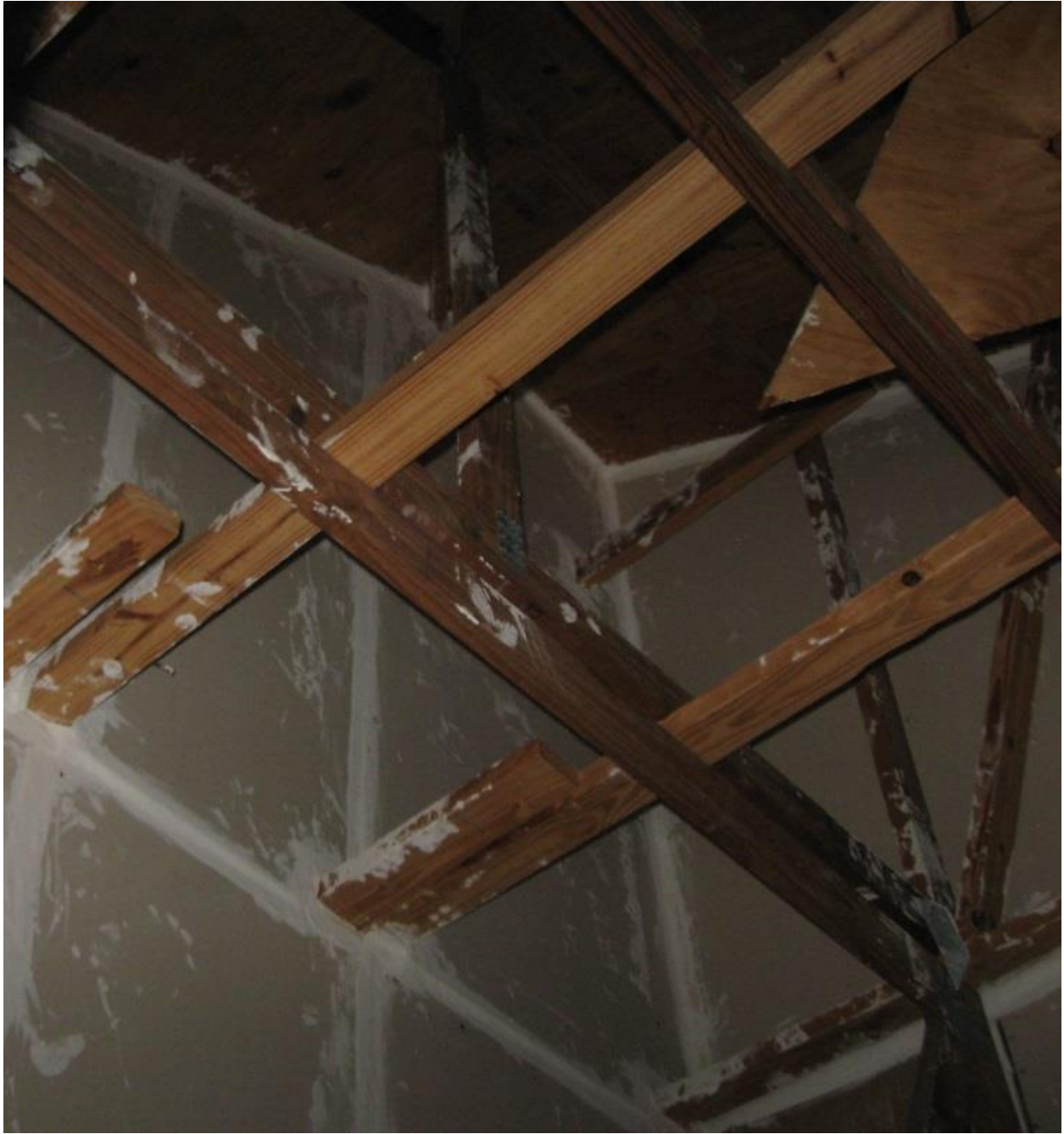
Picture 05 – Gypsum Draftstopping with All Penetrations and Joints Sealed with Mud and Tape
