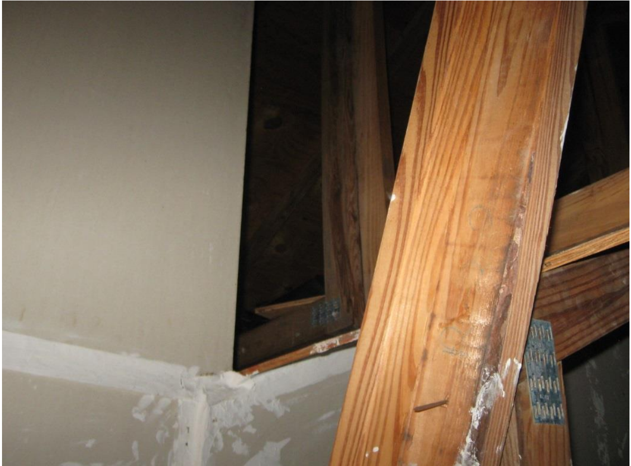
Picture 10 – Building 12 Deficiency.
