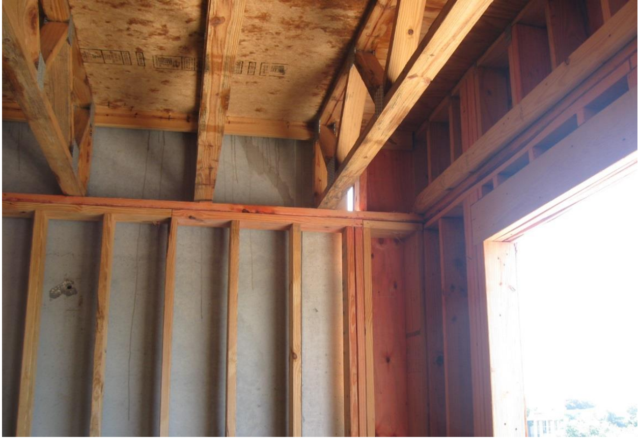
Picture 15 – Floor Terminating into Exterior Walls in Type III Construction with Exterior Walls of Fire-Retardant-Treated Wood at Concrete Fire Wall
