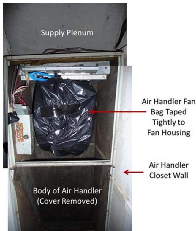
Figure 8. Return portion of air distribution system isolated from the supply by sealing around the air handler fan with a plastic bag taped at all edges.
