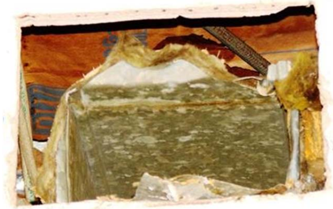
Figure 7. Disconnected supply duct
