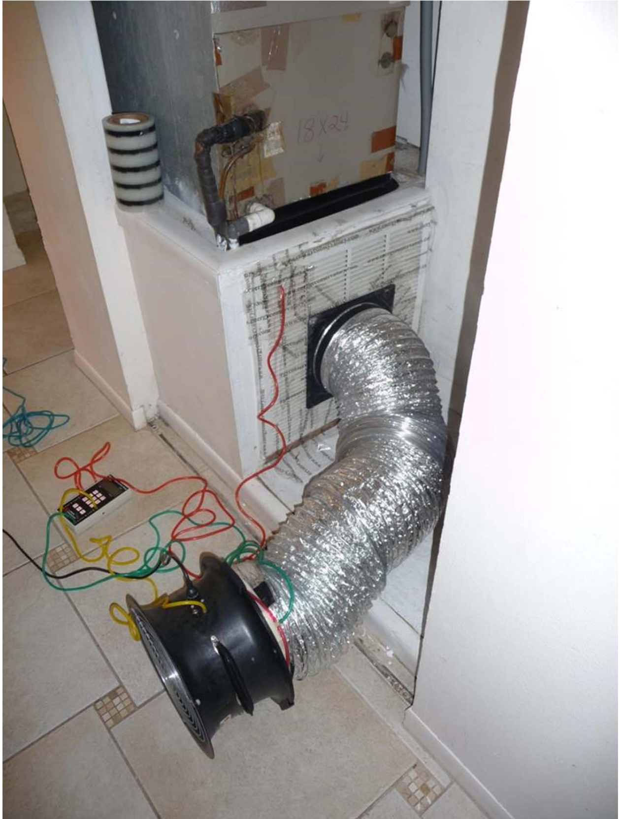
Figure 20 Pre-retrofit duct testing in progress
