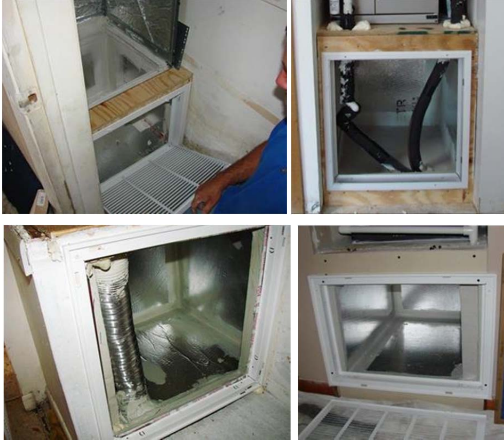
Figure 33. Air barrier lined return plenums in Test Houses (left to right) 1962, 194, 261, and 223.
