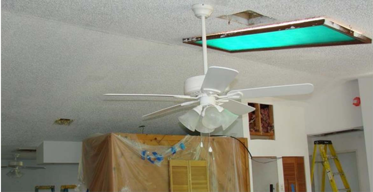
Figure 13. The hole in the wall over the air handler closet was cut to facilitate supply plenum installation. Also note the living room supply, to be relocated during repair.
