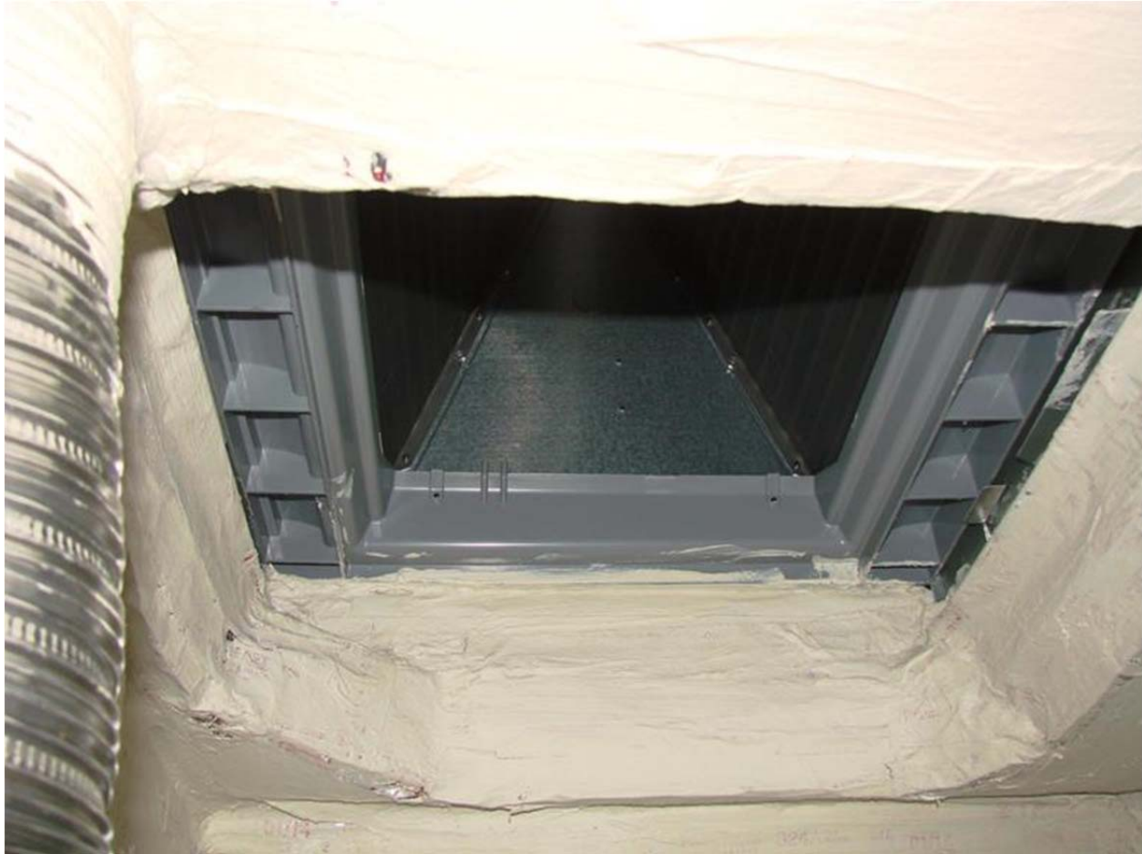
Figure 123. Return air entry to air handler seen from inside the return plenum. Joint between plenum, platform, and air handler is thoroughly sealed with mastic.
