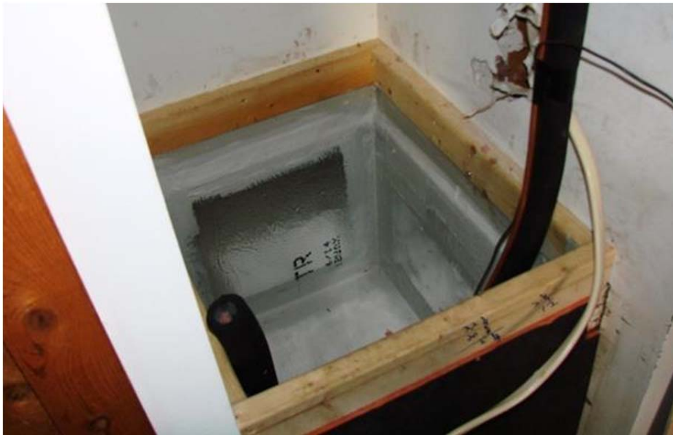
Figure 14 New duct board lining provides an air barrier to separate the return air stream from adjacent open wall cavities.
