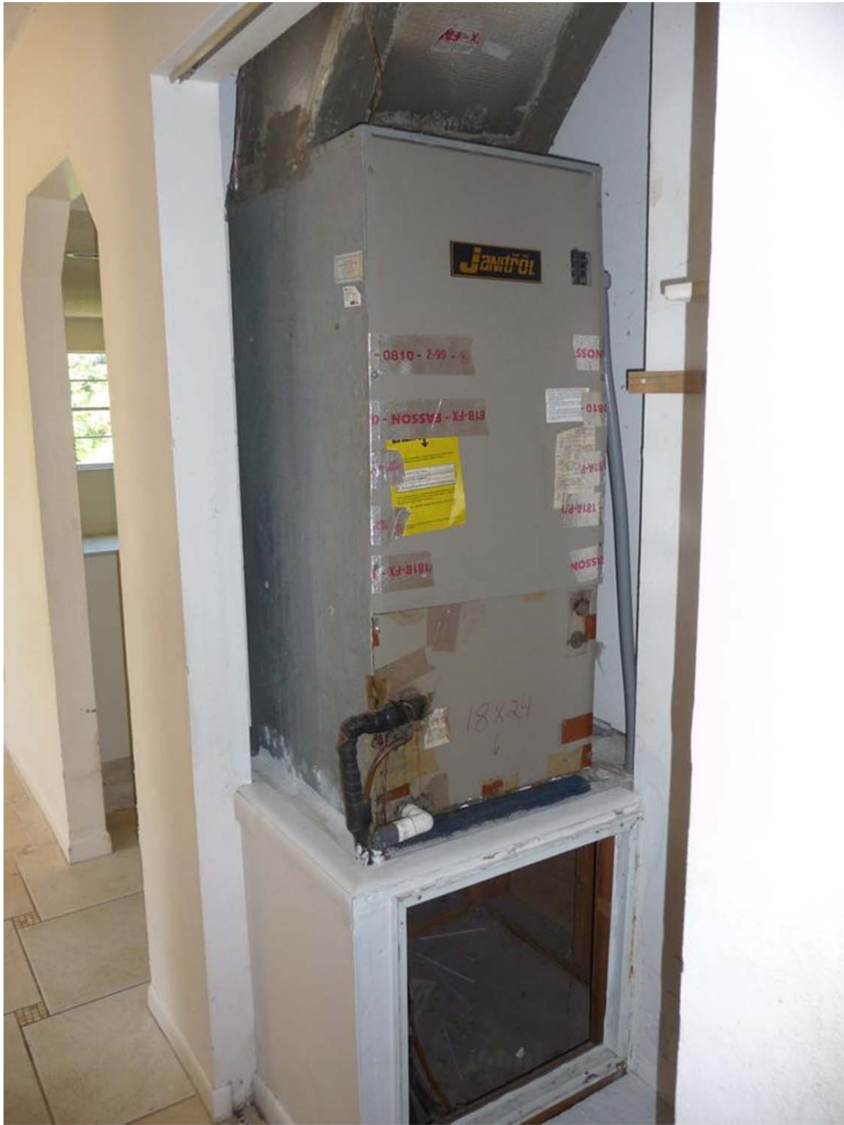
Figure 18. Note the open wall cavities in the return plenum and the raised plywood floor in the closet (in the lower right corner of the image)
