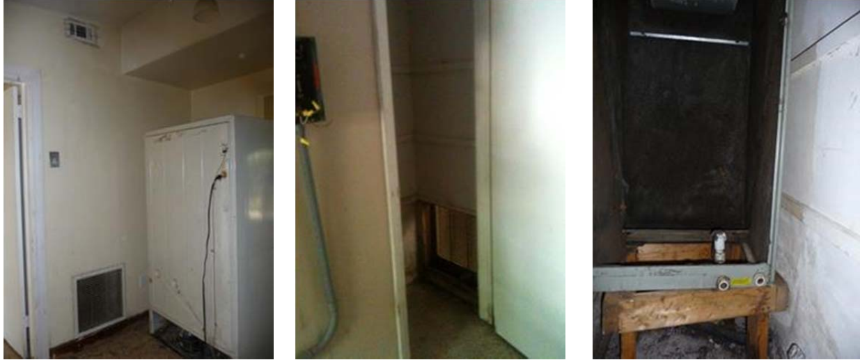
Figure 5. The entire air handler closet serves as the return plenum. Left: Central (only) return air grille mounted in wall between kitchen and air handler closet. Center: Air handler closet showing back of return air grille. Right: Inside the air handler closet, to the left of the door, showing air handler mounted on free-standing wooden supports.
