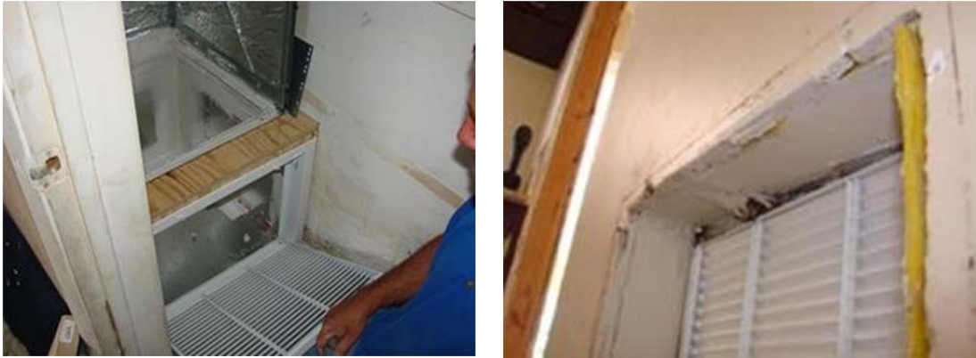
Figure 9. Filter-back return grille installed on new platform return in existing air handler closet (left). Air barrier blocking air flow down common wall (right).
