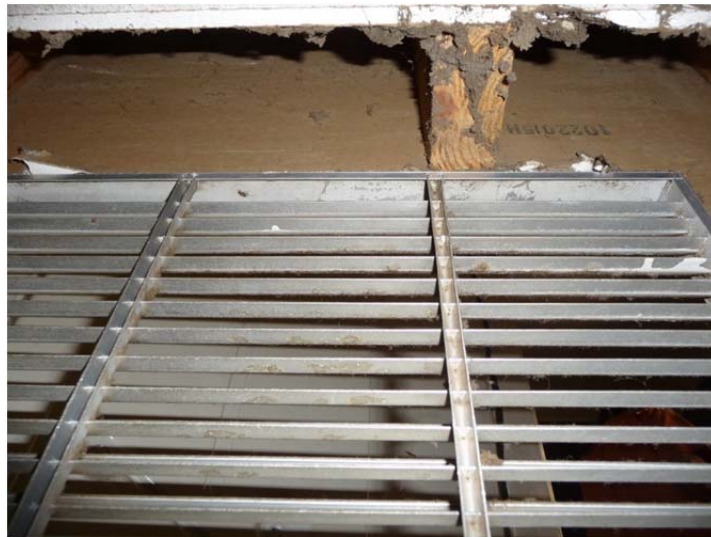
Figure 6. Looking up into the wall cavity from the wall-mounted return air grille. This wall cavity is part of the return air plenum because there is no air barrier separating it from the return air flow path.
