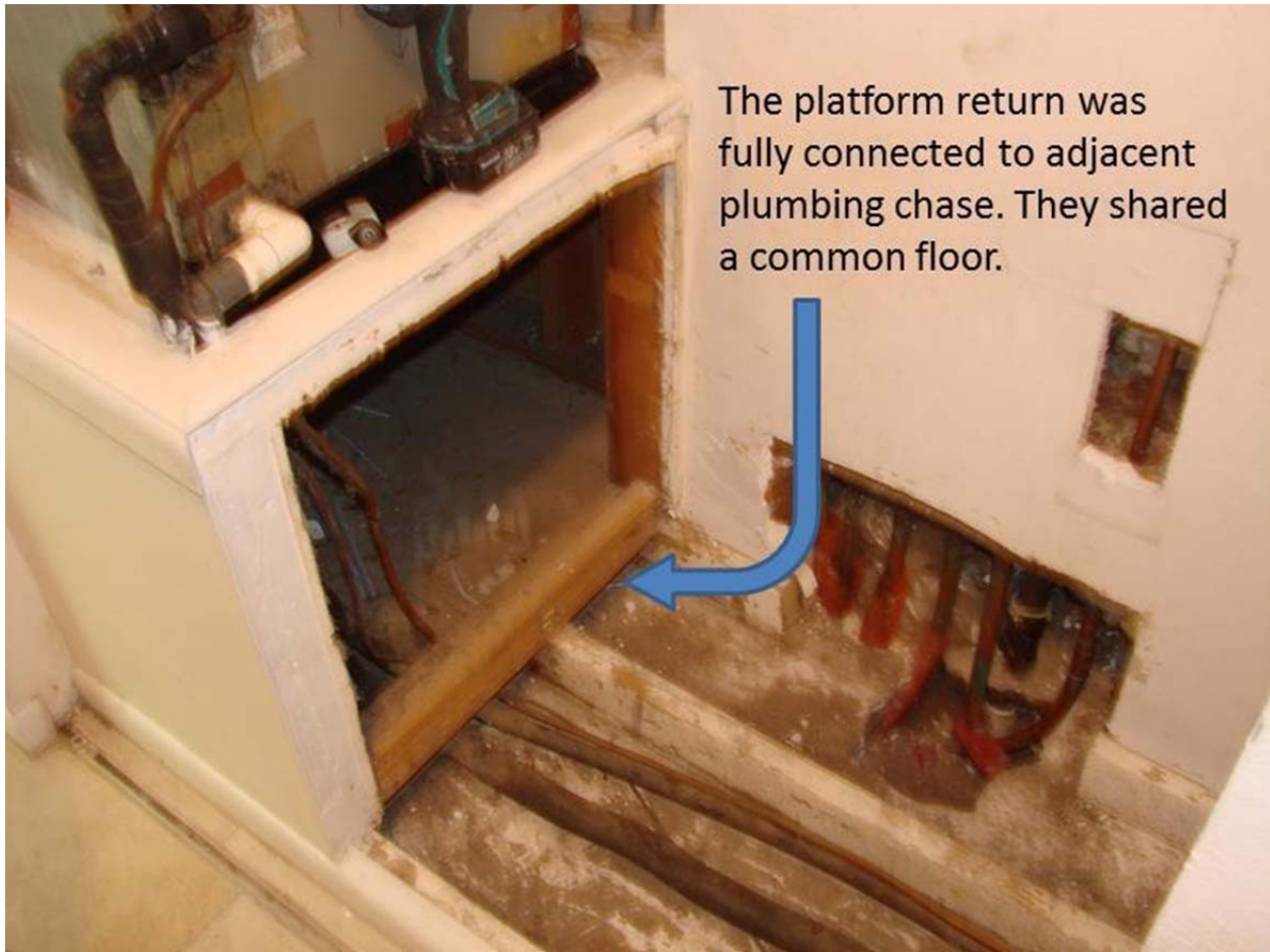
Figure 19. Raised closet floor created a plumbing chase for refrigerant line, condensate drain line and other plumbing runs. Chase is fully connected to return air plenum at pipe penetrations.
