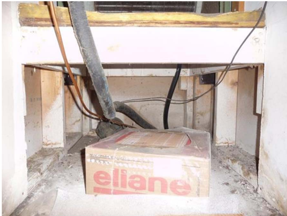
Figure 27. Open frame platform return.
