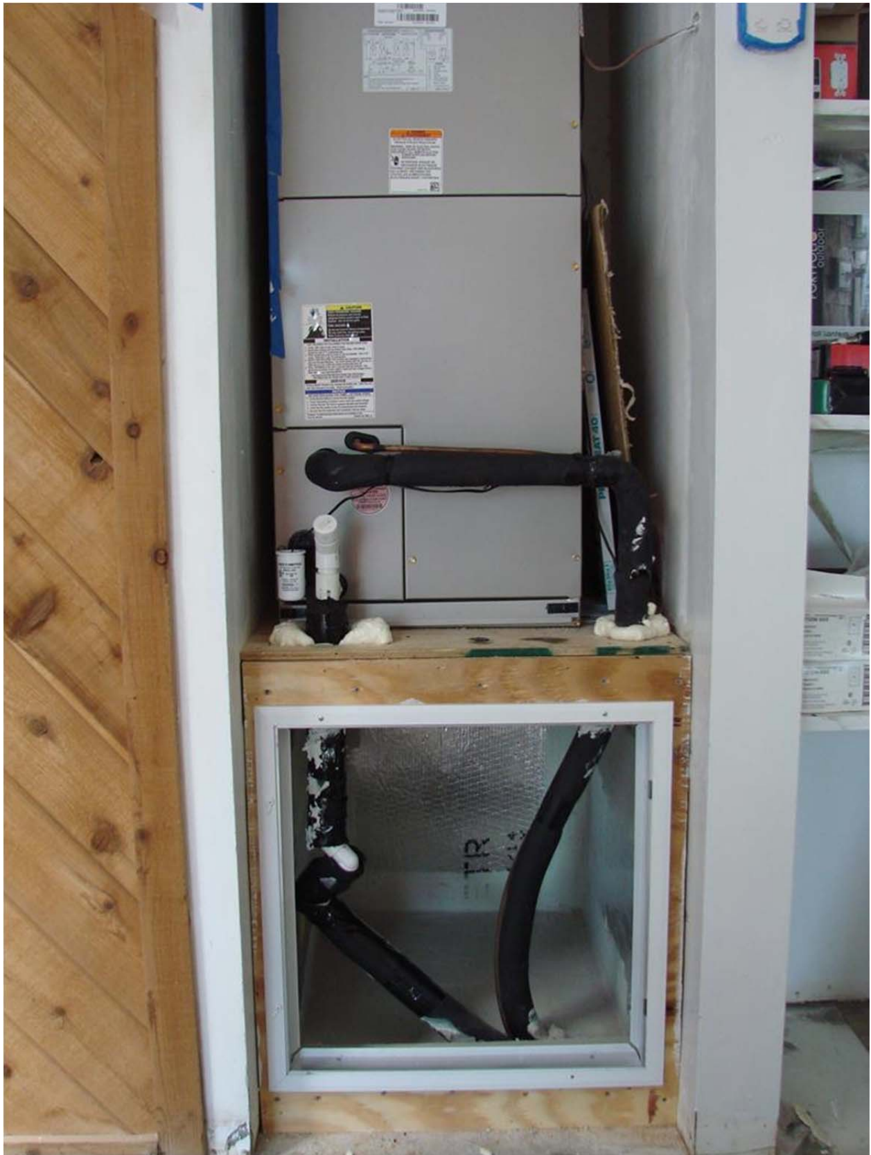
Figure 15 Completed repaired return air plenum. Note mastic at duct board seams.
