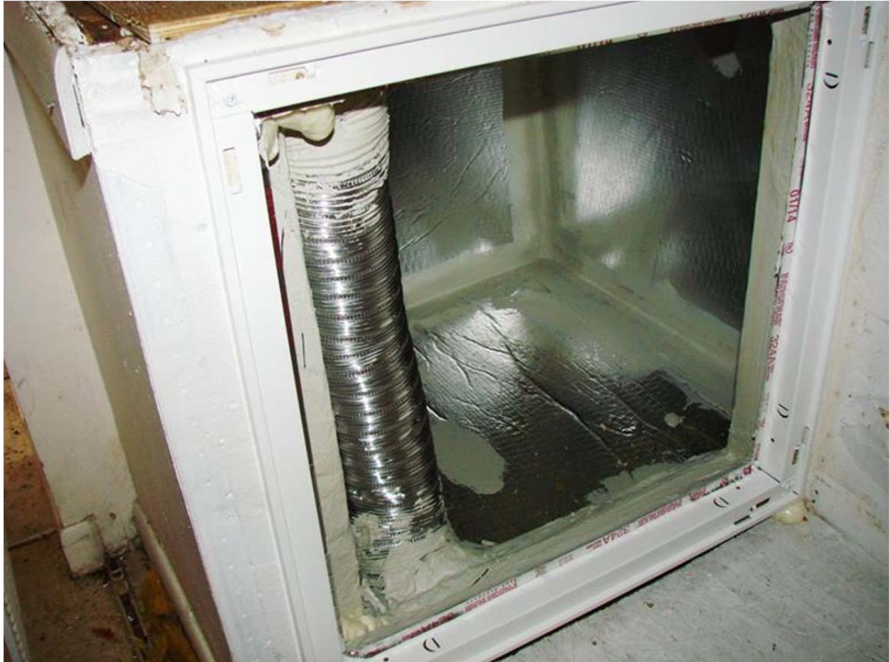
Figure 22. Repaired return plenum lined with duct board air barrier sealed with mastic at all edges.
