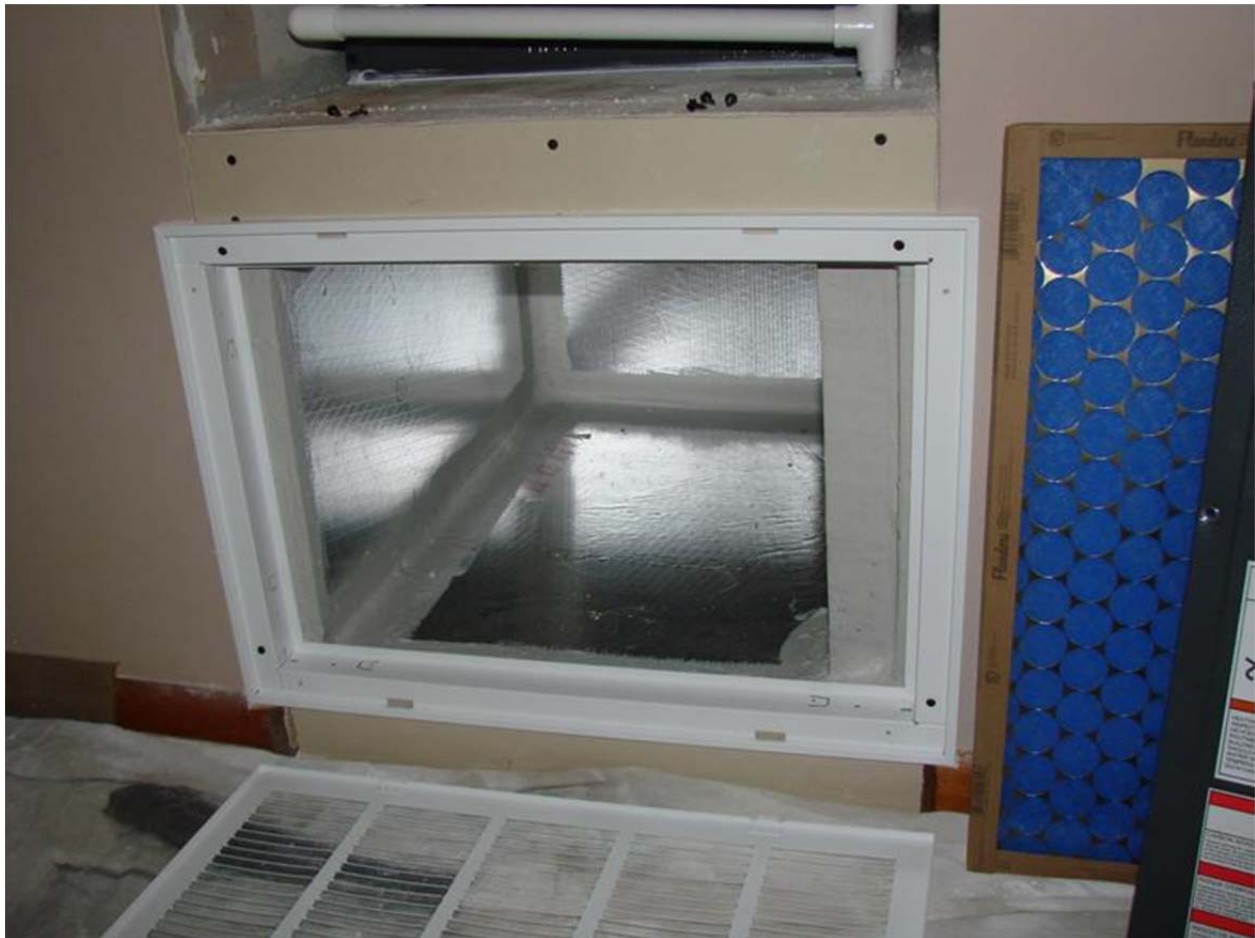
Figure 28. Repaired platform return plenum with duct board air barrier sealed at edges.
