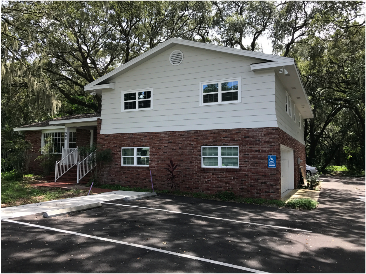
Front Exterior of building.
