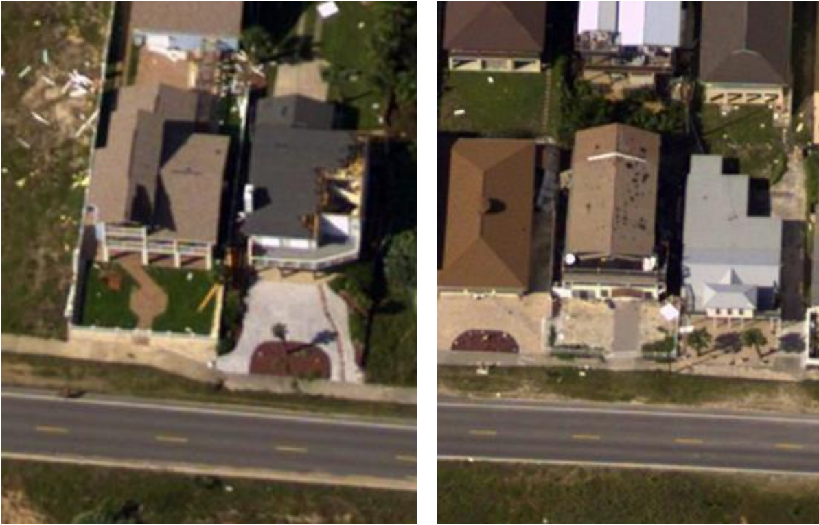
Figure 23: Examples of roof structure damage (left) and roof cover damage (right) visible in the aerial photographs provided by FCDEM.
