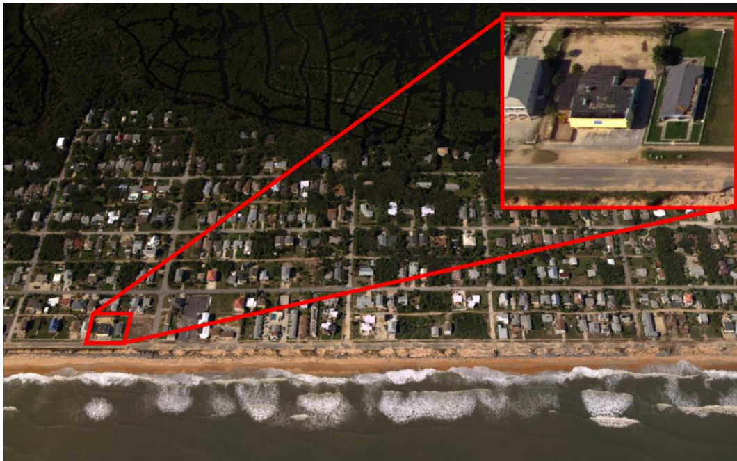
Figure 22: Photo “2016obP28253668.jpg” from a database of aerial photographs provided by the Flagler County DEM, with inset showing zoomed in view of roof sheathing and shingle damage to a multi-family home (far right of inset) at 1908 S Ocean Shore Blvd. Damage ratios for roof cover and roof sheathing were estimated to be 15%.
