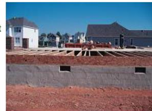
Vent openings in a stem wall foundation provide cross ventilation
