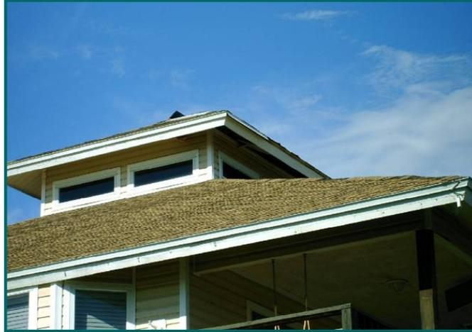
Composite shingle roof—some hip/ridge loss.
