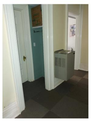
Photo 11 – Level 2 Water Cooler Non-Ada Compliant
