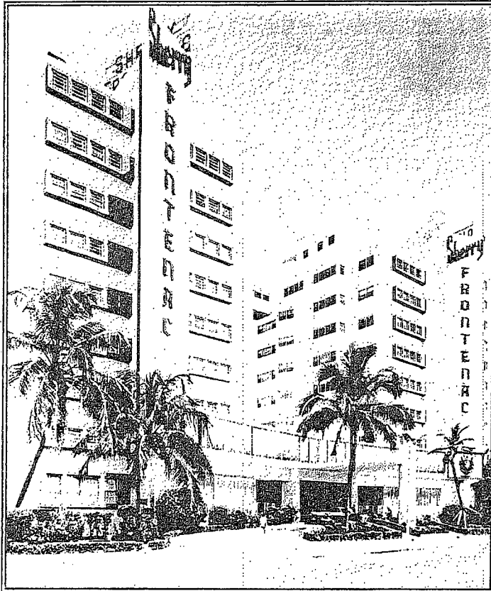
Figure 24 The fabulous Sherry Frontenac Hotel, located at 6565 Collins Avenue, was designed by Henry Hohauser in the Post War Modern style in 1947. The hotel featured twin nine-story towers that were connected by a central three-story lobby. The saw-tooth shaped plan of the twin towers provided many of the hotel rooms with views of the ocean and allowed for maximum sunlight. The Sherry Frontenac Hotel offered their guests many amenities, including an expansive lobby that overlooked the ocean, a dining room with a mezzanine level orchestra pit, a night club, an Olympic-sized pool, and private beach cabanas. Guests were greeted with a sweeping portecochere when they arrived at the hotel.
