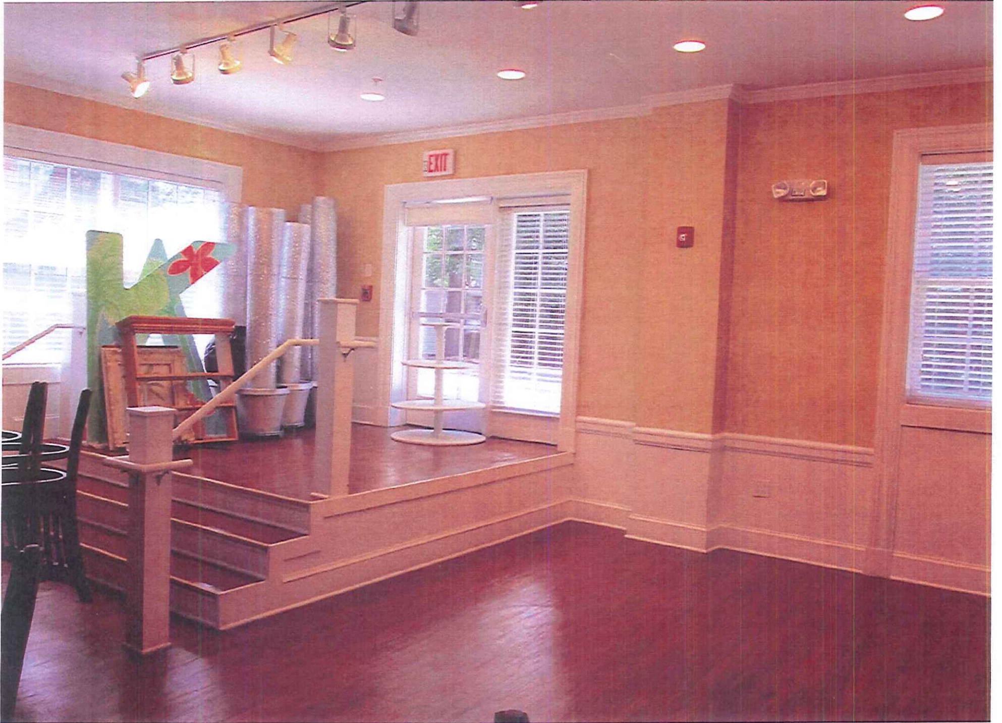
Second Exit Platform from Dining Room
