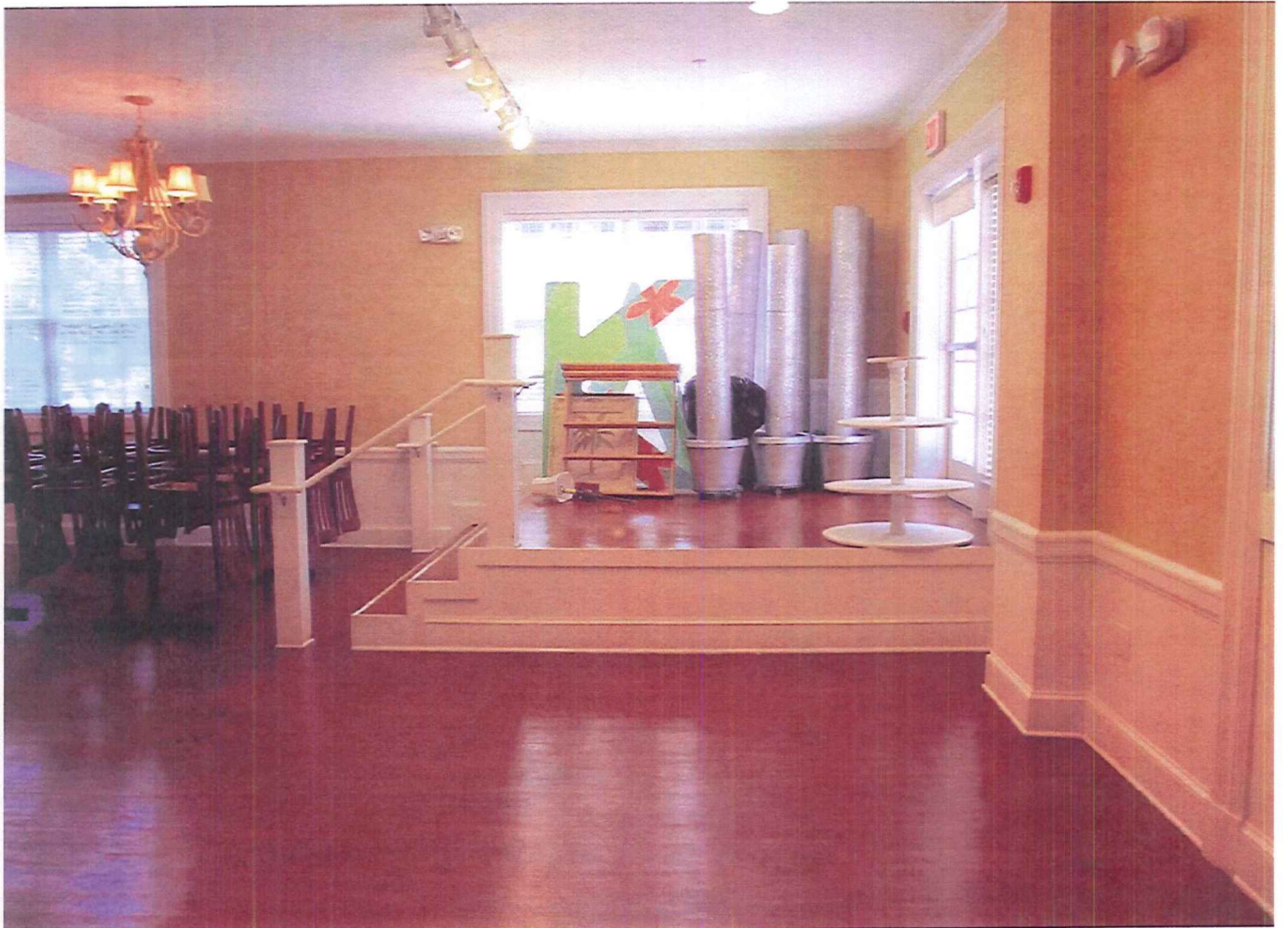
Second Exit Platform from Dining Room
