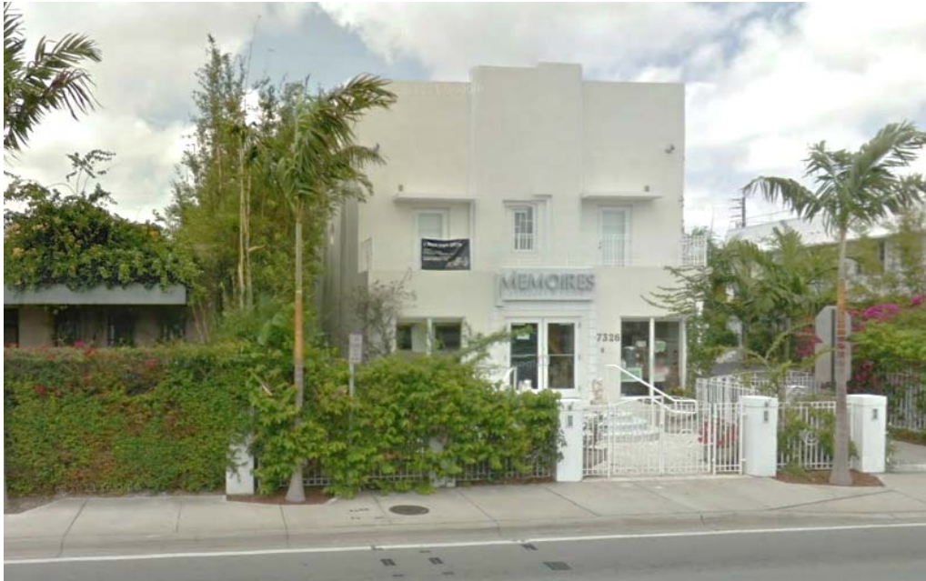
7320 BISCAYNE BLVD NORTH PROPERTY LINE VIEW
