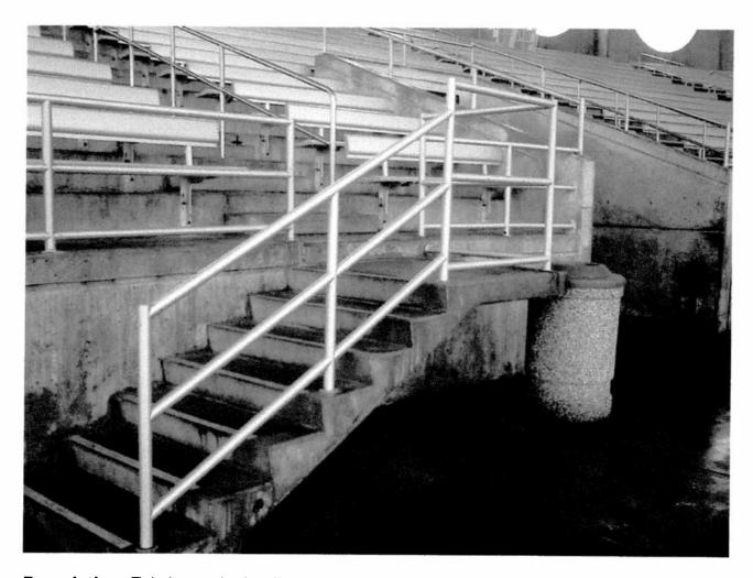
**Description**: Existing stairs leading to the upper grandstands' aisle stair along the middle accessible aisle. The upper grandstands are approximately 36 inches above the middle accessible aisle to enhance viewing.
