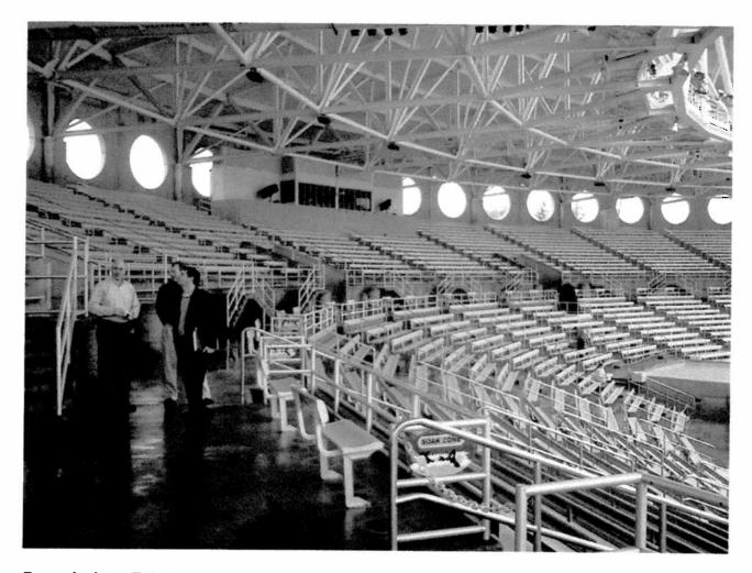
**Description**: Existing middle accessible aisle continuous between upper and lower grandstands and serves as a means of egress to each accessible space. Each module between aisle stairs at lower grandstands provides 4 accessible spaces + 4 companion spaces as indicated on this photo. There are 64 existing accessible spaces along this middle aisle, with *many lines of sight*.
