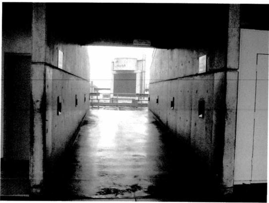
**Description**: Existing sloped, accessible means of egress route (bottom photo is tunnel) from vomitory. This route leads to middle accessible aisle between upper and lower grandstands and serves as a means of egress to each accessible space. See Exhibit -2 for existing accessible spaces along middle accessible aisle.
