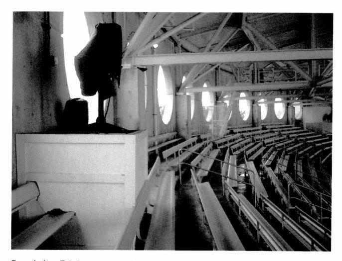
**Description**: Existing upper grandstands' aisle accessway (space between rows of seating). The existing space between each row is 2'-9" and 12 inches vertical rise. The clear aisle accessway space is 15 inches. The seating additions at each end will match the row spacing and seating of existing as shown.
