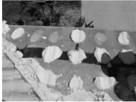
Problems with bond of tile to mortar and mortar to underlayment
