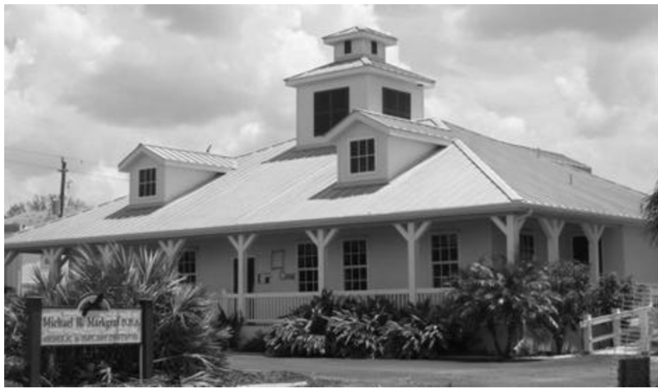
5 V-ribbed metal that did well...a lot of fasteners in this system
