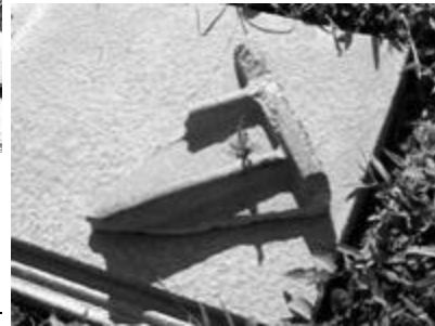
Flat tiles nailed with 0 to 1 nails
