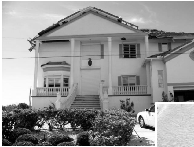
Soffit and framing damage
