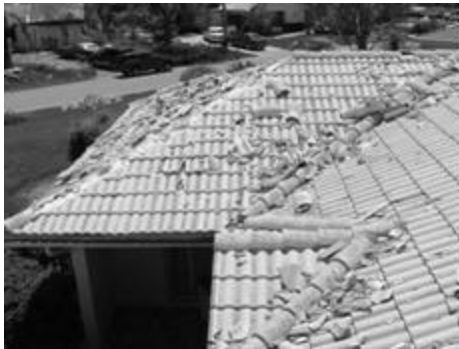
Problems with mortar at hips and ridges
