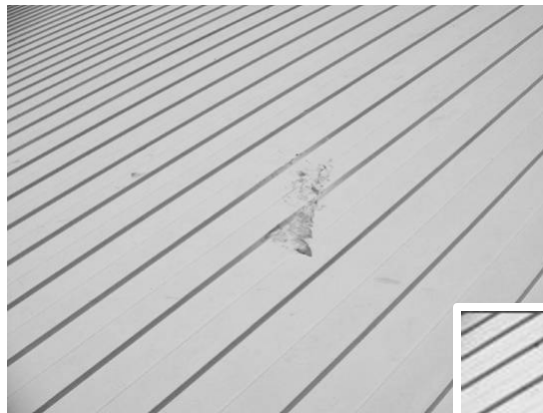
Scattered debris from adjacent roof
