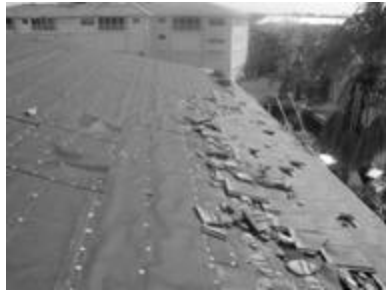
Mortar—wrong location
