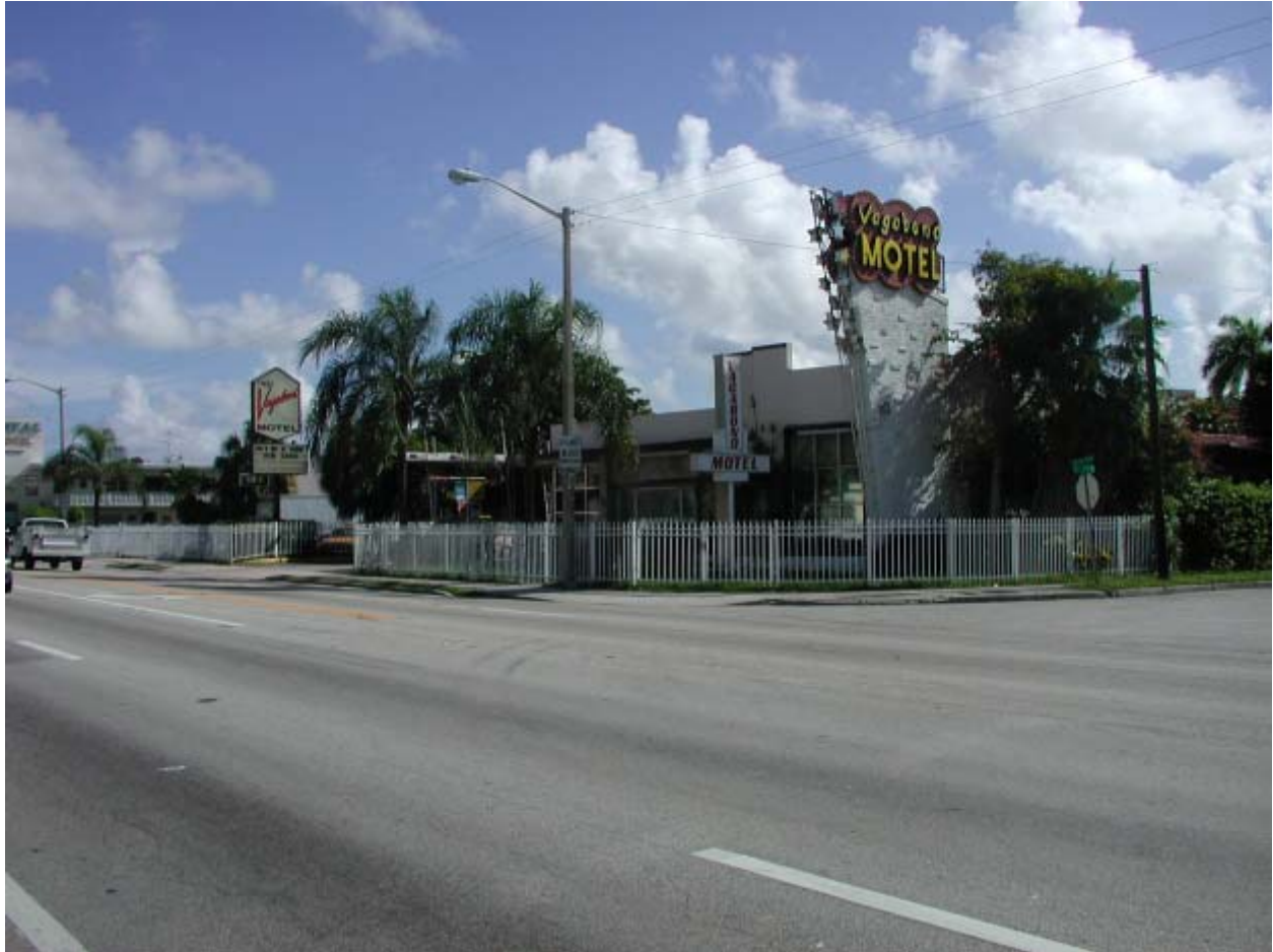
Figure 9. The Vagabond Motel 7301 Biscayne Boulevard, 1953 Miami Modern
