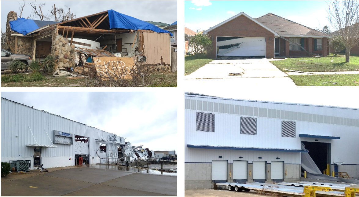
Figure 17. Illustrative large door failures; (top left) pre-FBC residential building in Mexico Beach area, (top right) post-FBC building in Panama City, (bottom left) pre-FBC commercial building in Panama City, (bottom right) post-FBC commercial building in Panama City.
