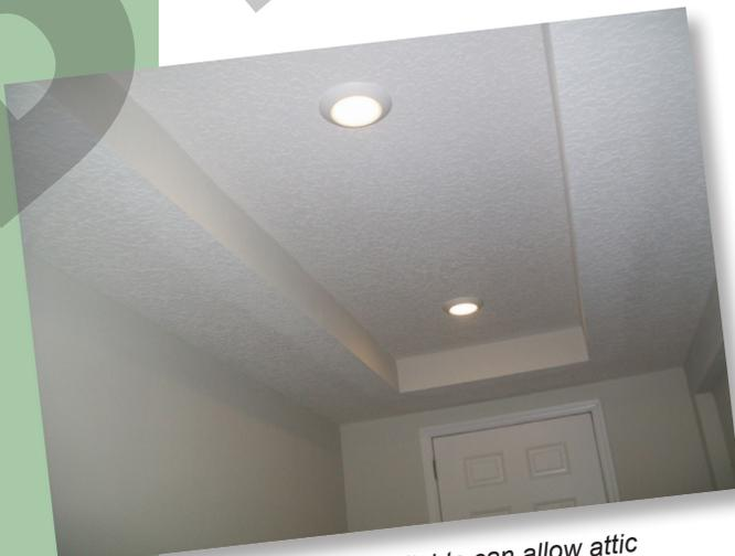
*Unsealed can lights can allow attic air to infiltrate into a house.*
