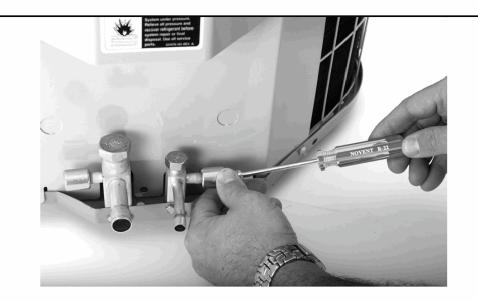
Figure 1101.10(1) INSTALLATION OF LOCKING CAPS FOR REFRIGERANT ACCESS PORT (Photo Courtesy of Novent LLC. & Airtec Products Corporation, Inc.)
