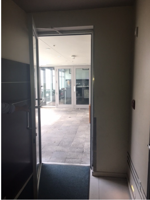
Pool access from lobby
