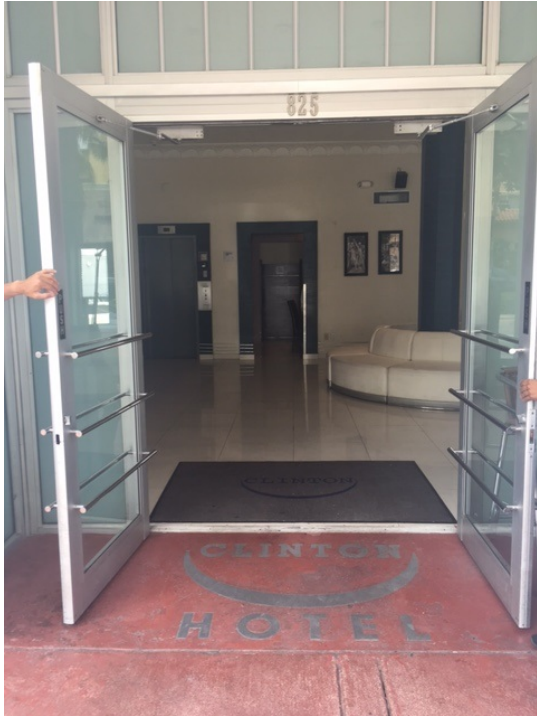
Front Entrance from Sidewalk
