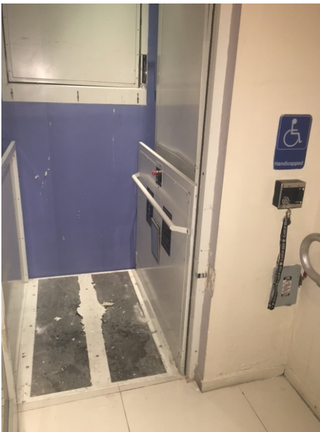
Handicap lift entrance
