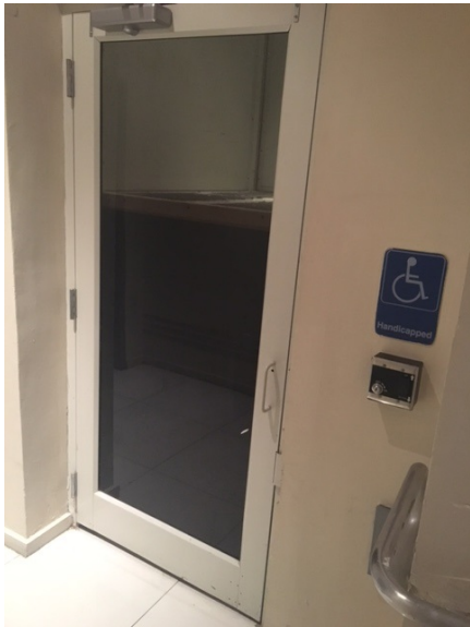
Handicap lift area to 1 st Floor
