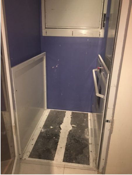
Handicap lift entrance
