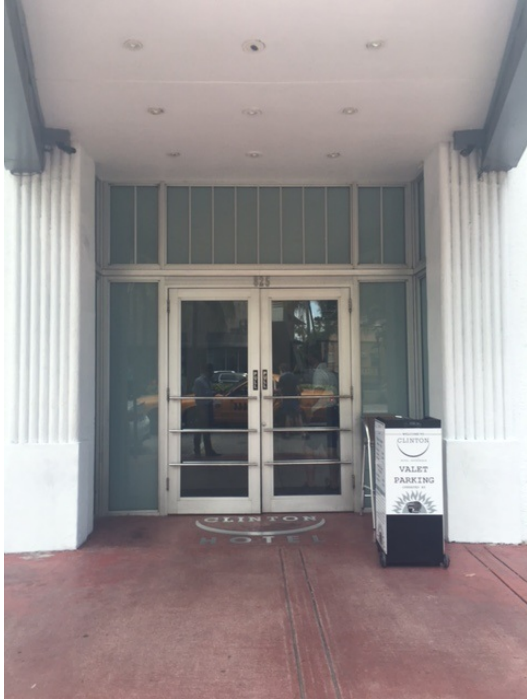
Front Entrance from sidewalk
