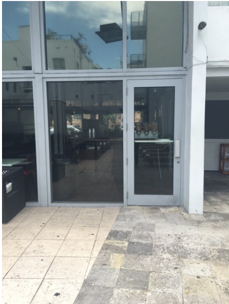
Pool deck looking into restaurant
