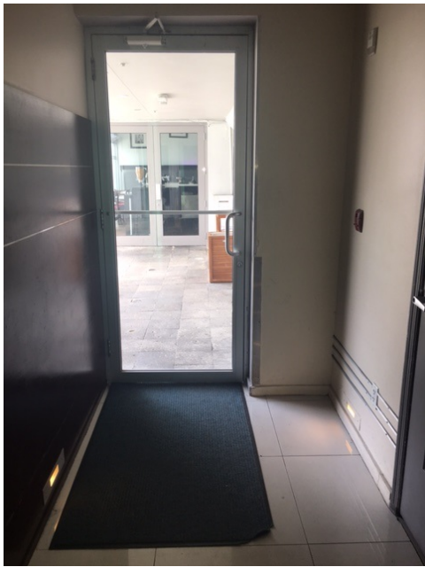
Pool access from lobby
