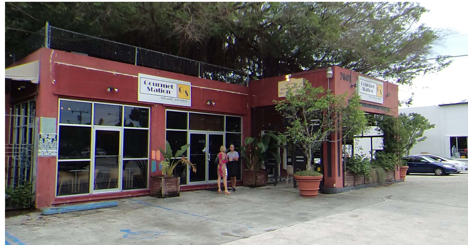
7601 BISCAYNE BLVD- NORTH NEIGHBOR (VIEW FROM BISCAYNE BLVD)
