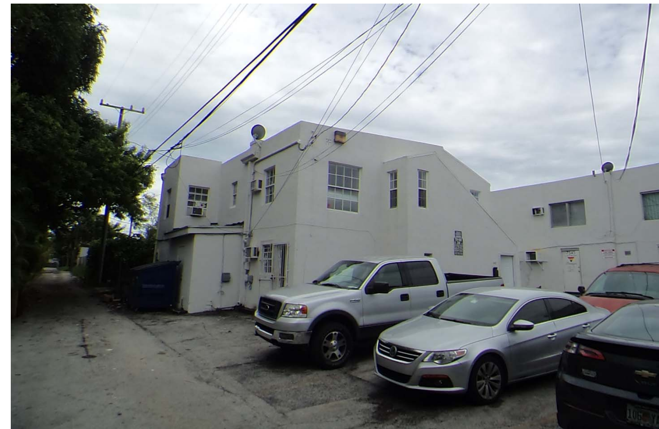
620 NE 76 th Street WEST PROPERTY LINE VIEW (ALLEY)
