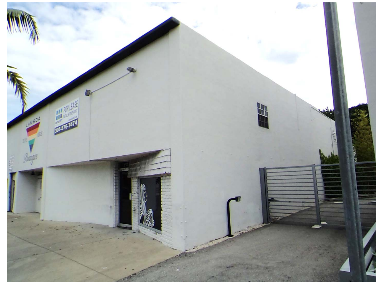
7541 BISCAYNE BLVD SOUTH PROPERTY LINE VIEW
