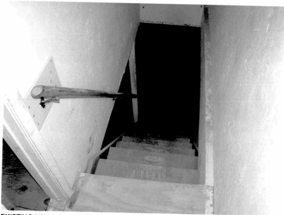
EXISTING MEZZANINE STAIR
