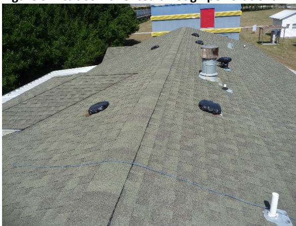
Figure 7. Attic off-ridge vent caps sealed.
