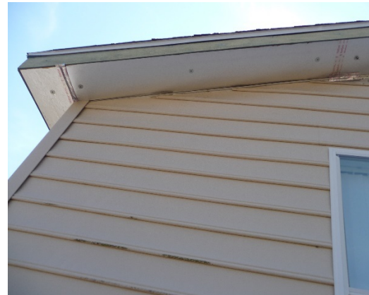
Figure 6. Attic soffit vents sealed.
