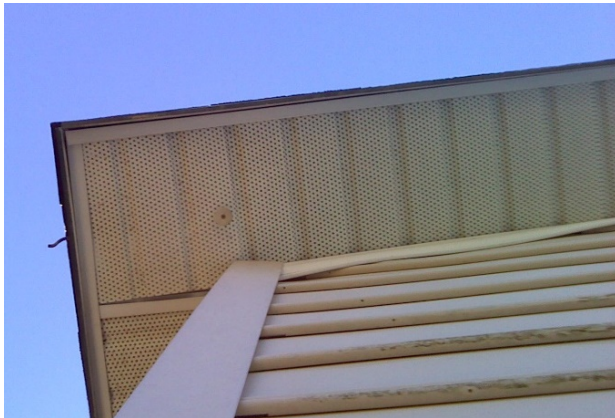
Figure 5. Attic soffit vented through perforations.
