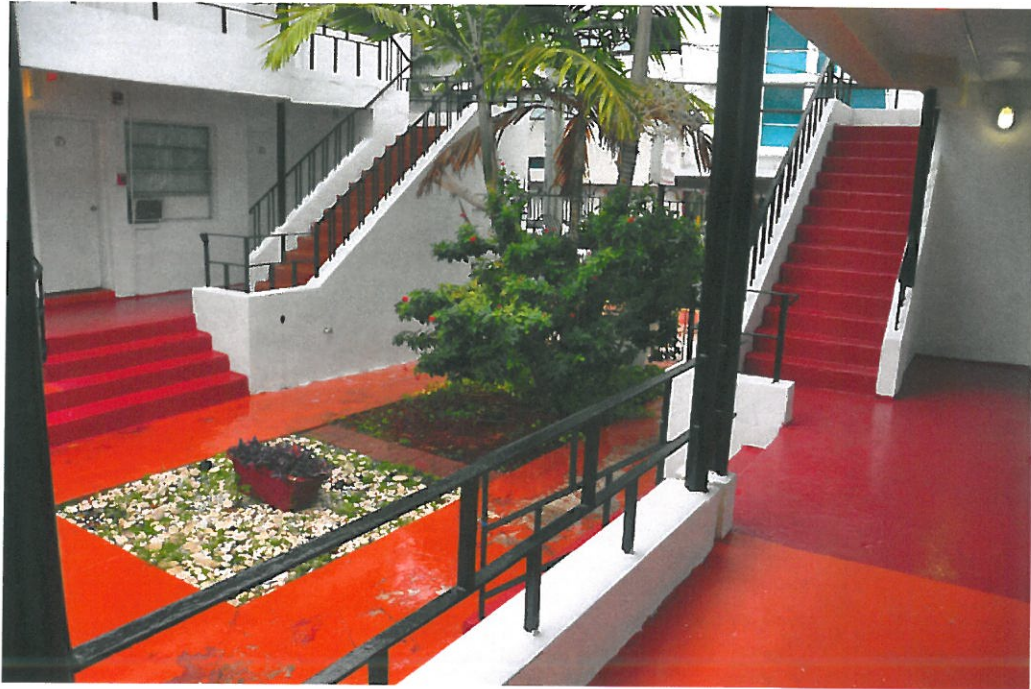
Courtyard entry, facing North
