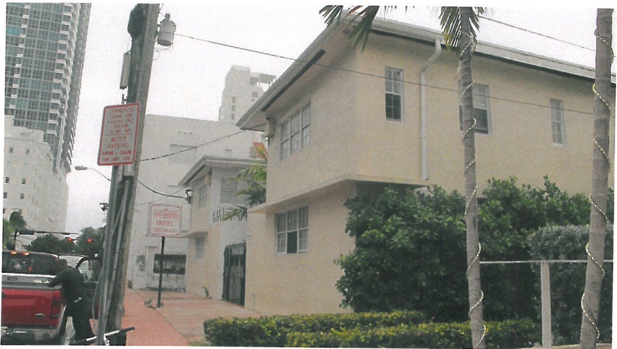
West facade and alley facing South
