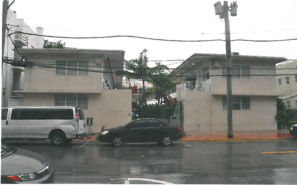
Front facade from 20th Street
