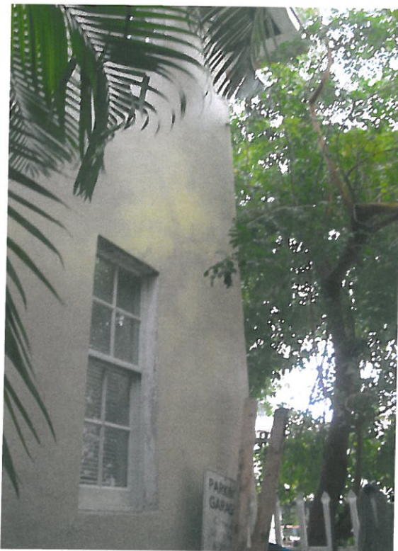
Southwest corner of building
