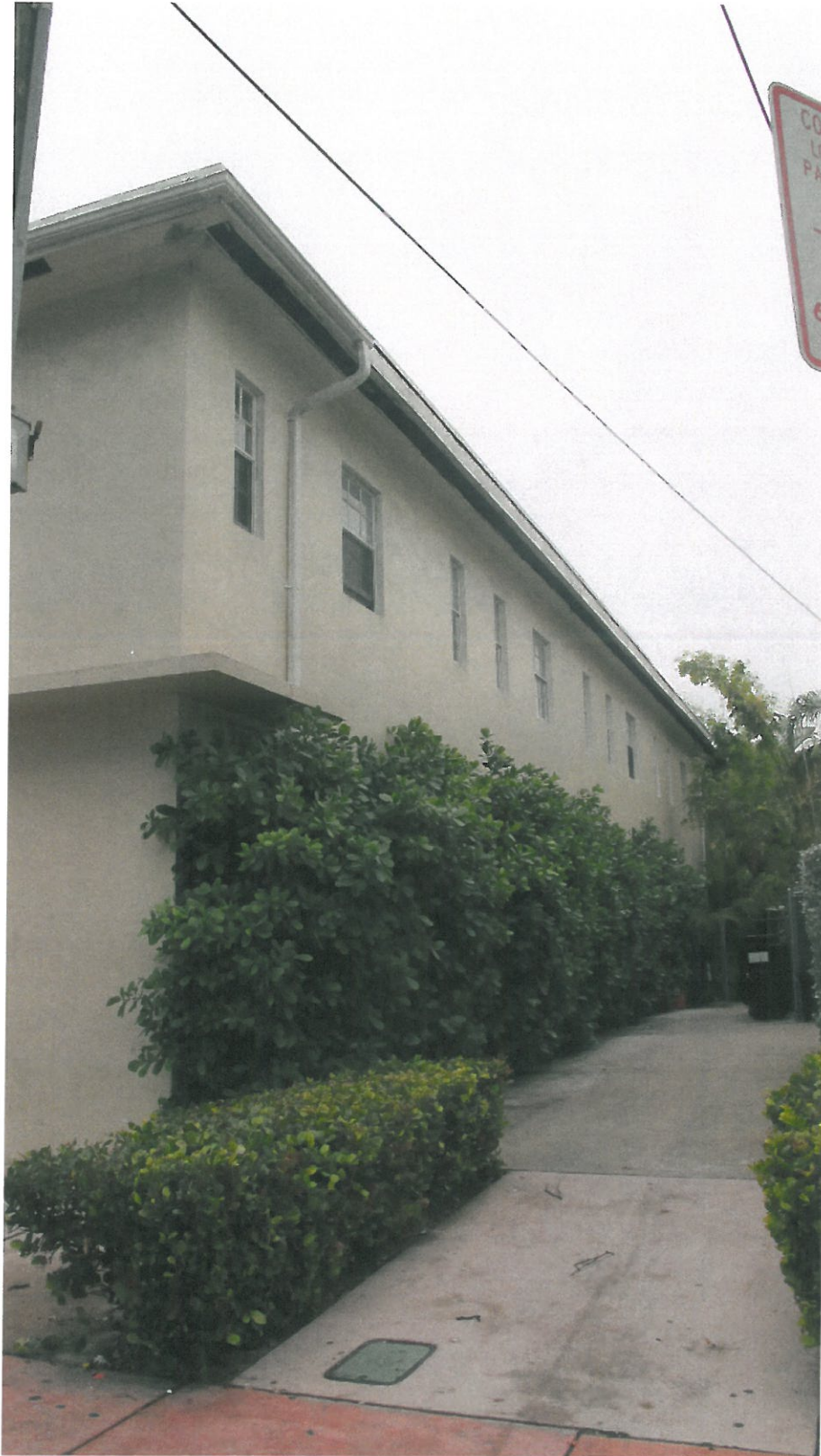
West side of North facade, facing Southeast
