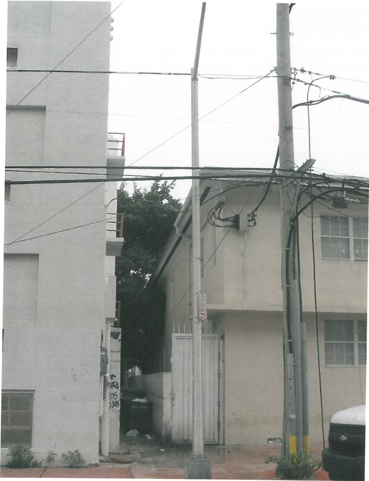
Northeast Corner facing South
