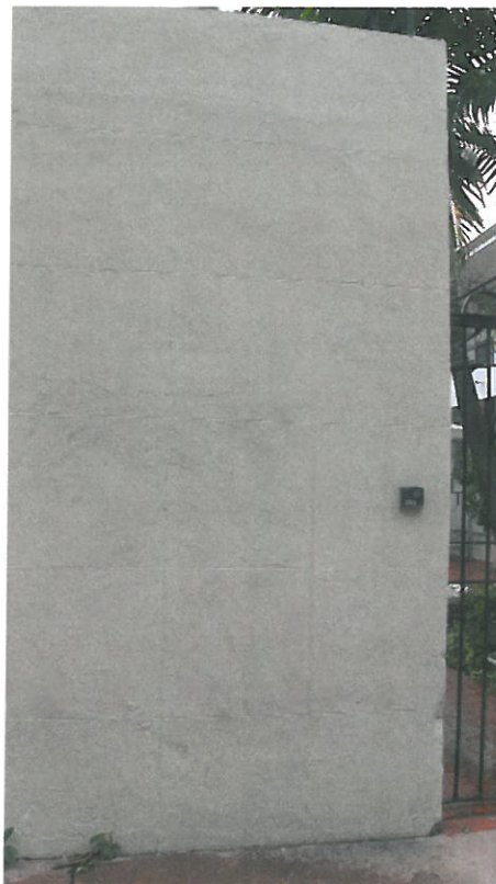
North facade facing South, Wall just East of Central Gate, with assumed historic grid pattern visible
