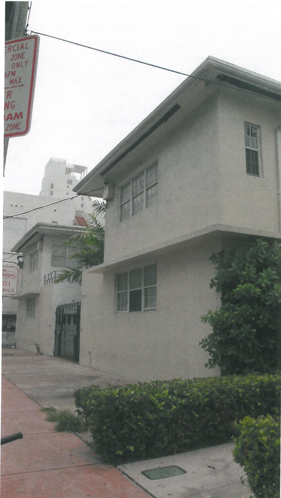
North facade and sidewalk, facing Southeast
