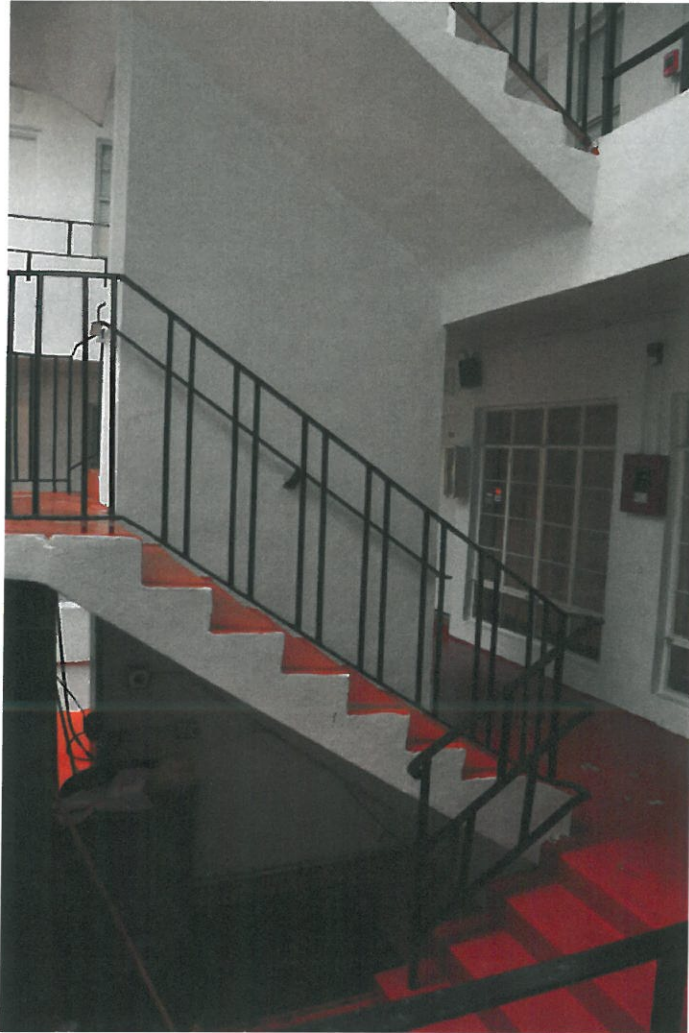
Central South Stair, facing East
