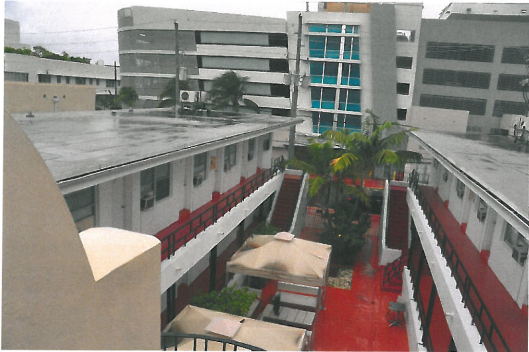
Courtyard from 2nd floor roof of front building
