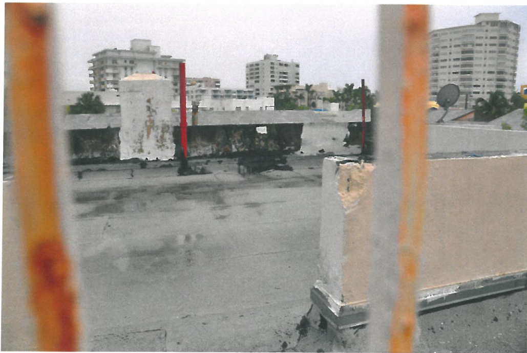
Roof on South side of building
