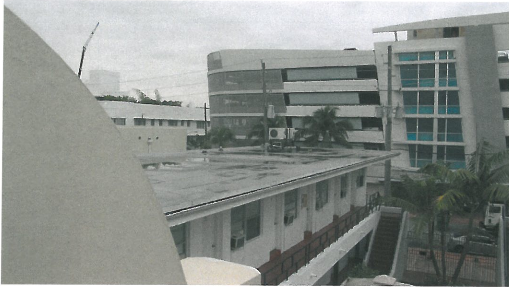
Roof of West building, facing Northwest
