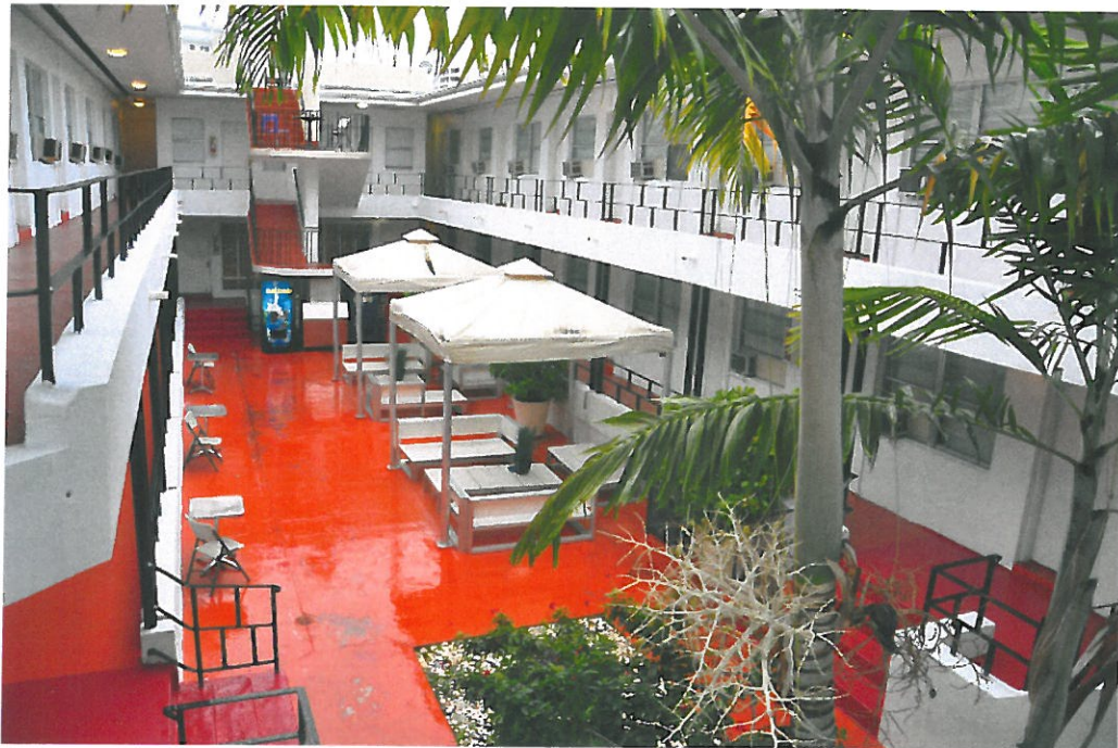
Central courtyard from Northeast stair, facing South
