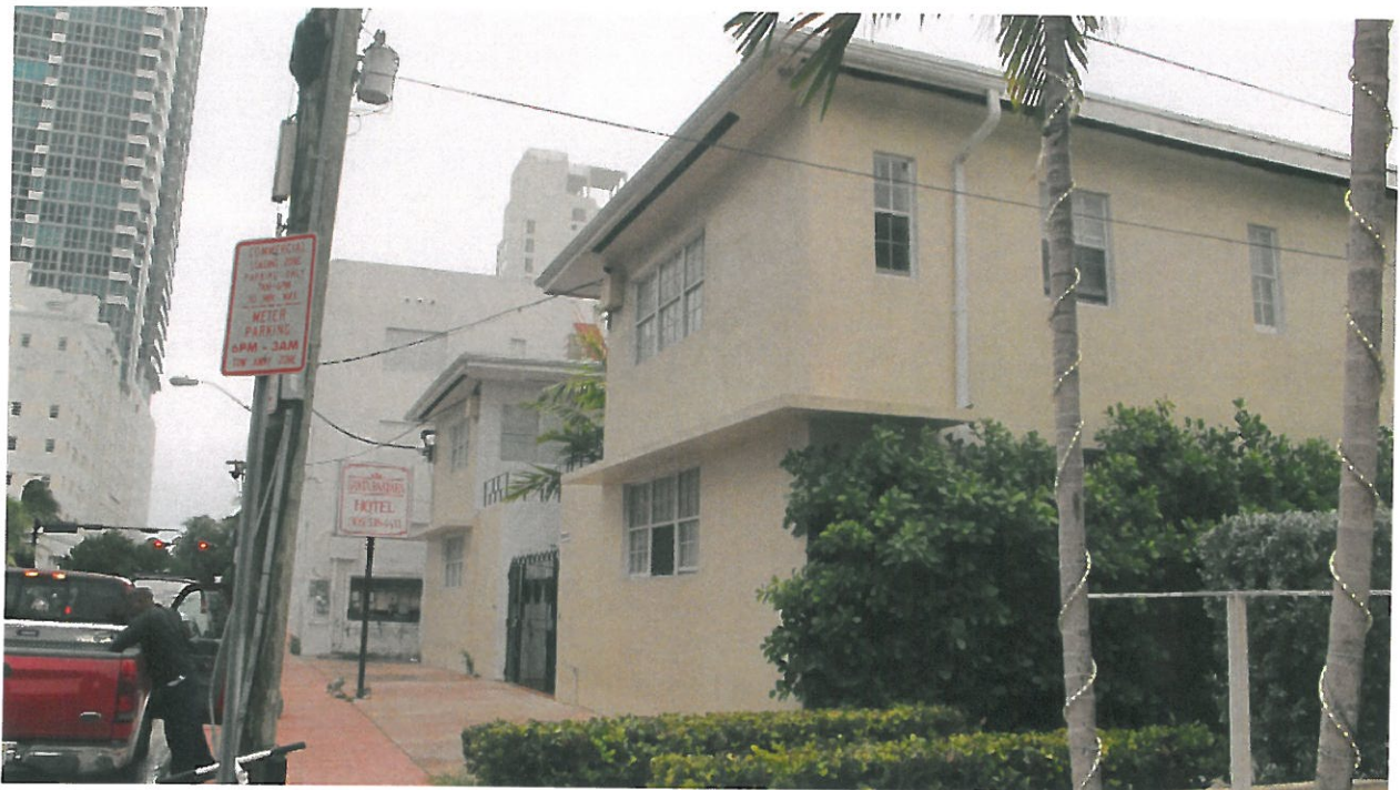
West facade and alley facing South
