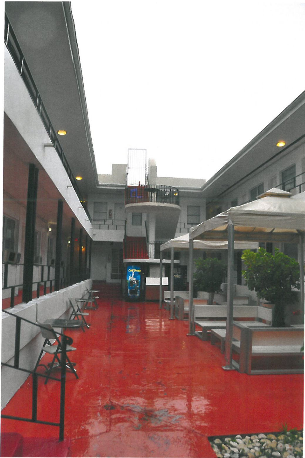
Central courtyard, facing South
