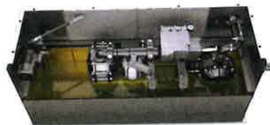
PUMP UNIT IN ELEVATOR PIT
