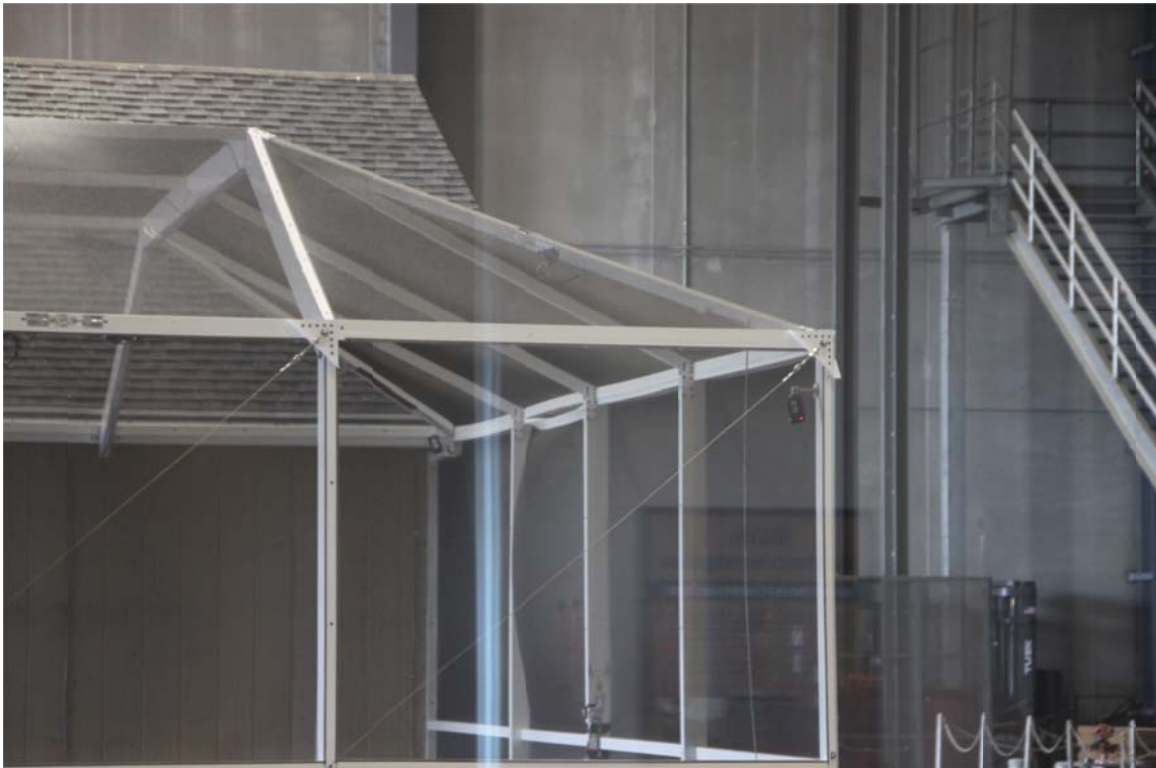
Figure 16. Partial failure of the screen attachment during Run 27 (maximum wind speed = 80 mph)
