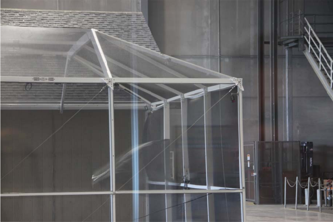
Figure 19. Failure of the screen attachment during Run 30 (maximum wind speed = 90 mph)
