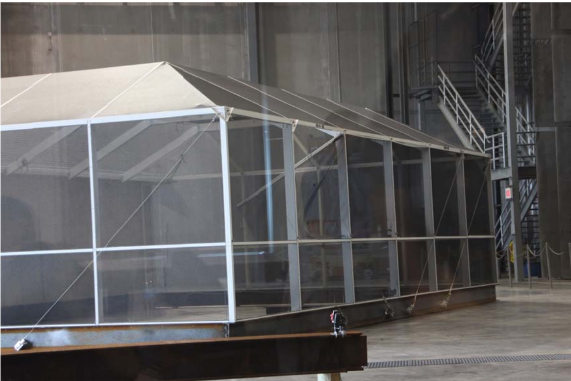
Figure 18. Failure of the screen attachment during Run 29 (maximum wind speed = 90 mph)
