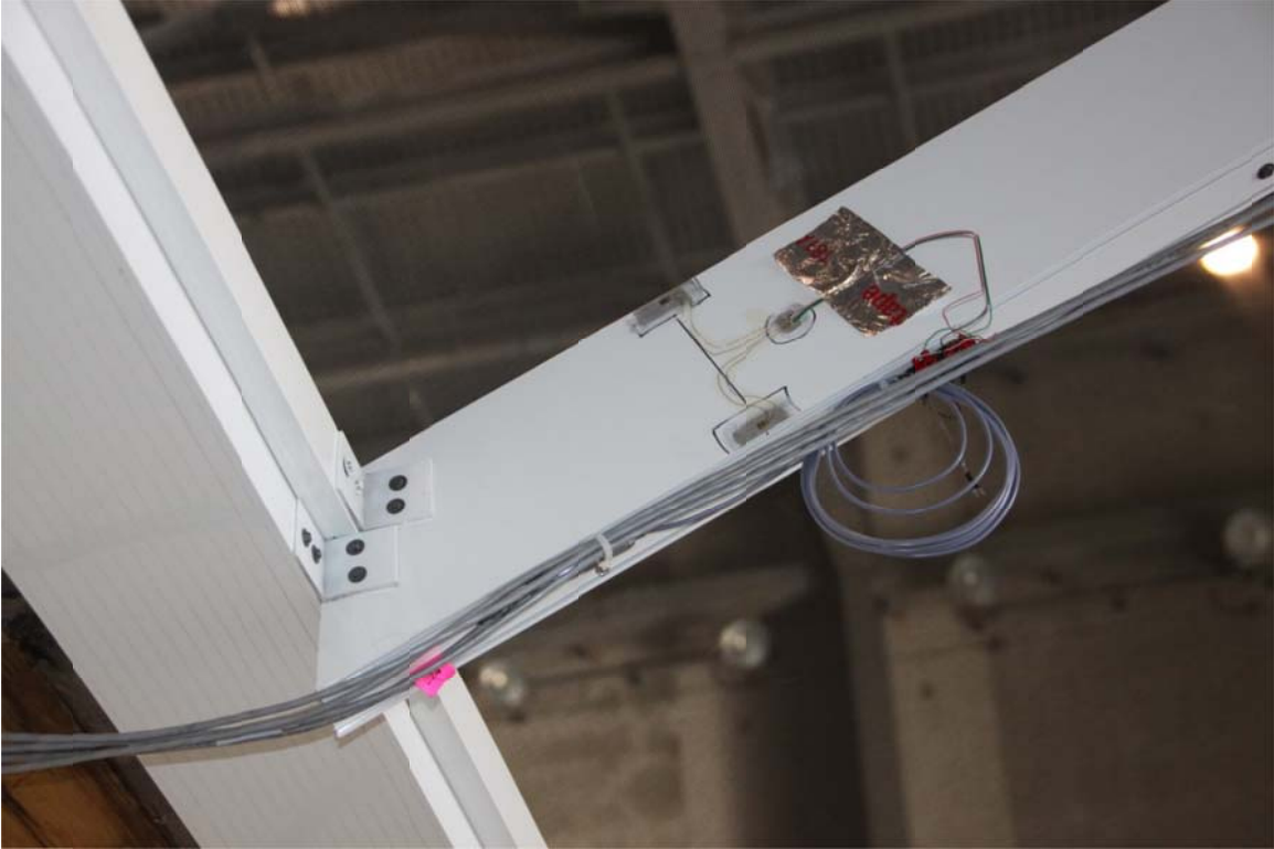
Figure 9. Strain gauges installed in a beam to measure the moment
