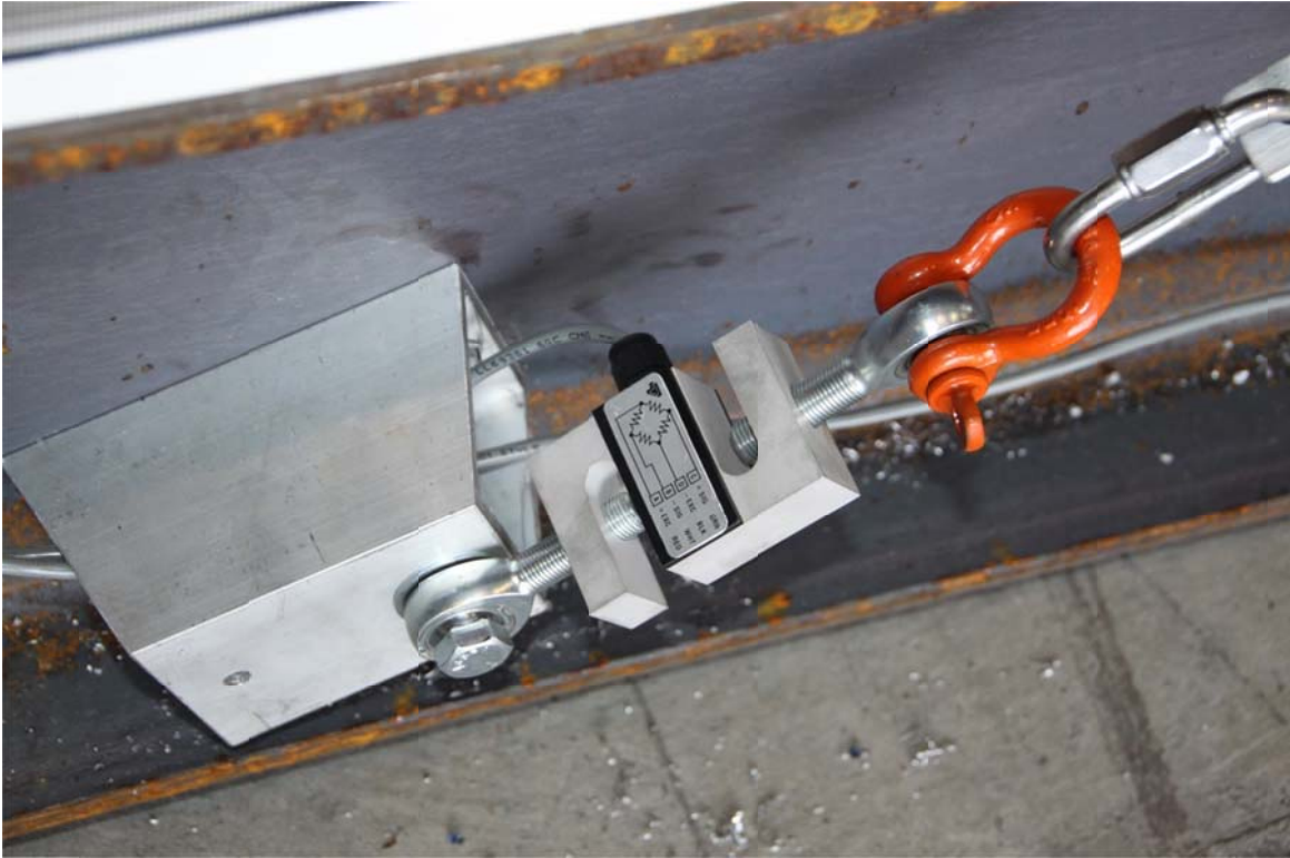
Figure 8. Load cell measuring the cable tension
