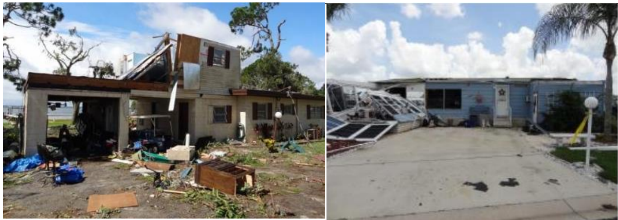
Figure 12: Post-2012 Lake Placid (Highland County) tornado damage showing EF2 damage (left) Post-2012 Vero Beach (Indian River County) tornado damage showing EF1 damage (right)
