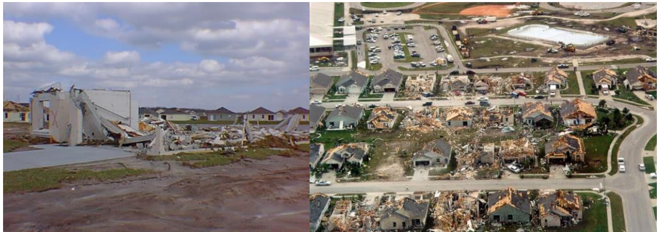
Figure 11: (Left) A destroyed concrete block and stucco home in Kissimmee, FL during 1998 F3 tornado ( http://www.srh.noaa.gov/mlb/?n=kissimmeepics ), (Right) Damaged homes in Lakeside subdivision in Kissimmee, Florida. The 1998 F3 tornado moved from the upper right to the lower left, narrowly missing a school. ( http://www.nws.noaa.gov/os/assessments/pdfs/cntrfl.pdf )
