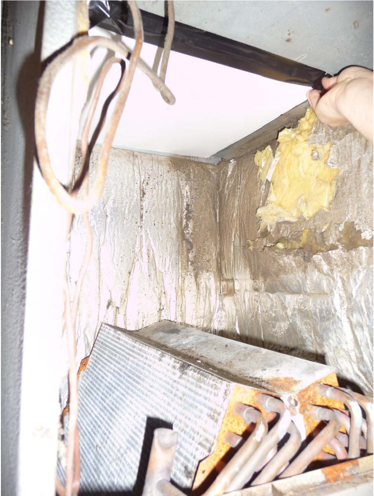
Figure 21 Blocking the supply side of the air distribution system for testing.
