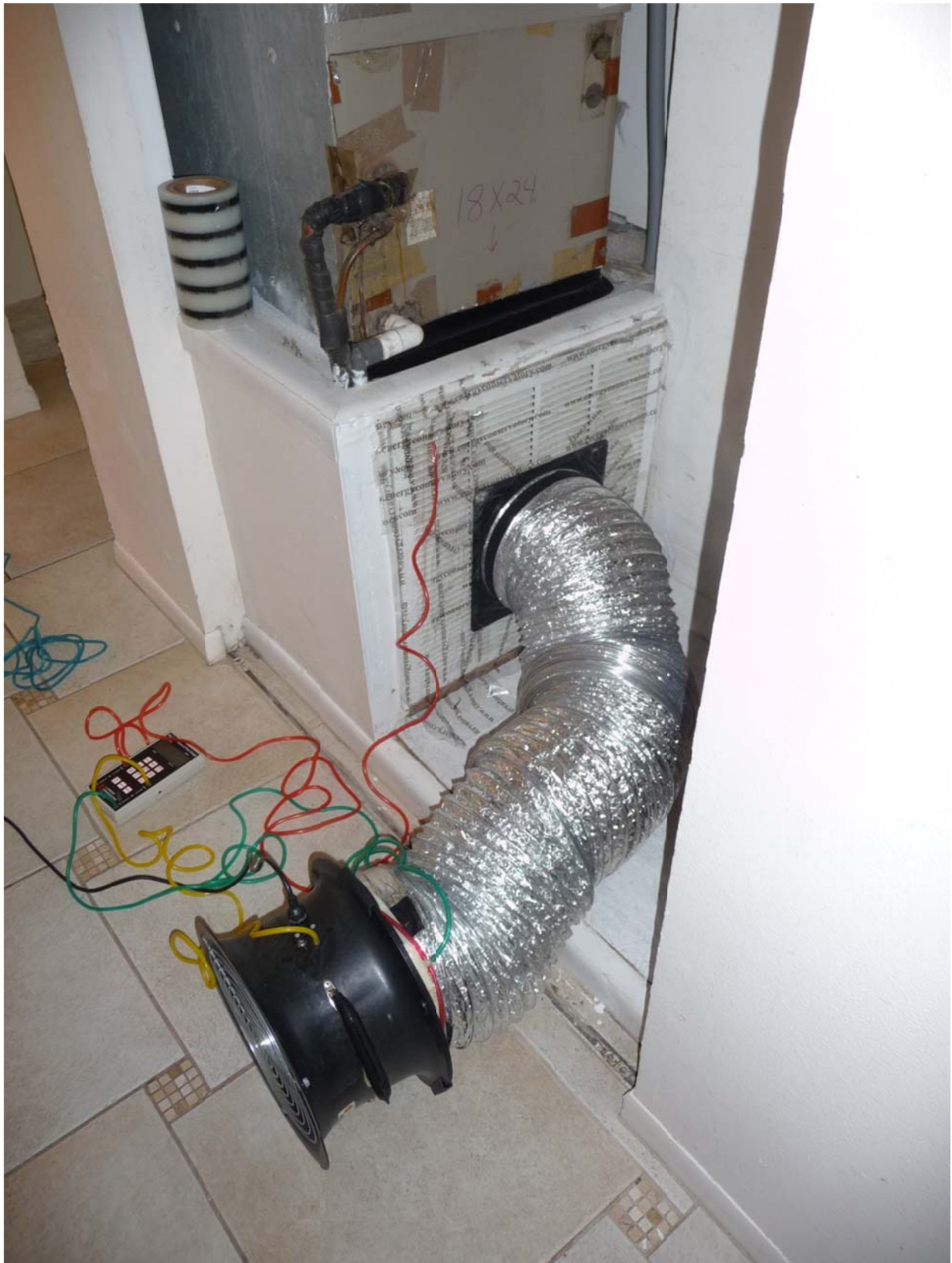
Figure 20 Pre-retrofit duct testing in progress
