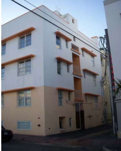
7 NW corner of building looking at alley
