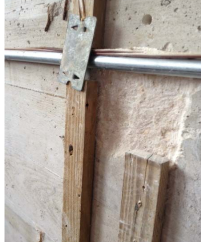
27 Reinforced concrete walls surrounding inaccessible space
