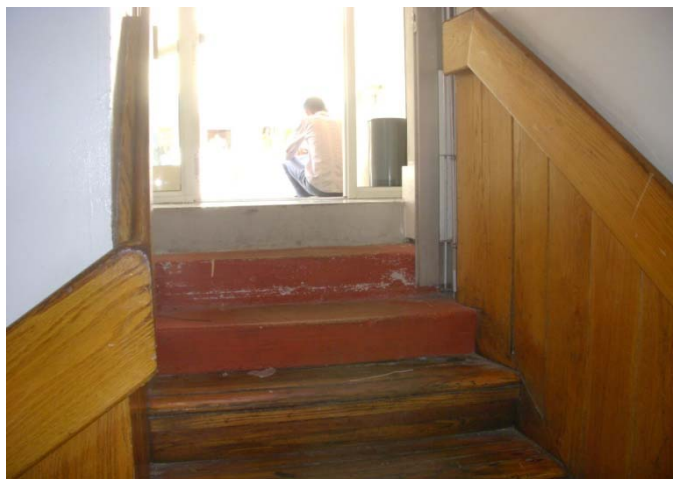
18 Looking up stairway to exit
