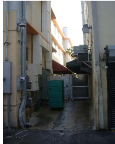
10 Building alley looking east / Accessible route gate entrance to main building
