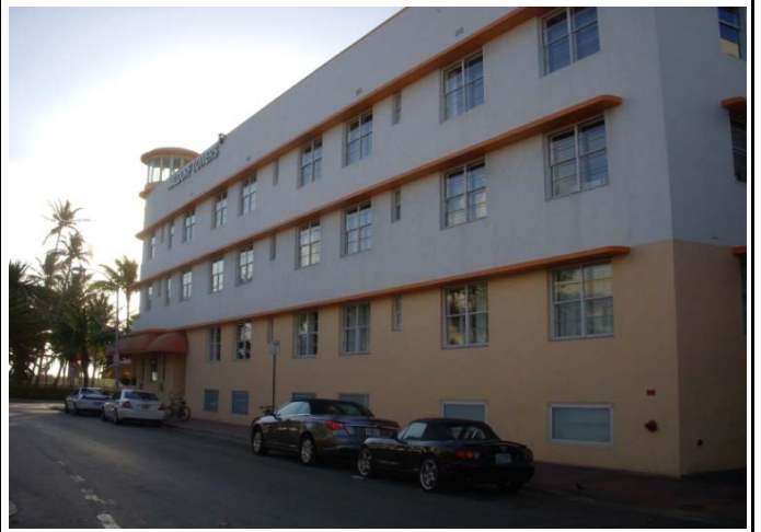
6 Exterior photo looking east down 9th Street
