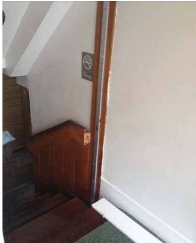
14 Stairway to proposed 7-11 space, with concrete walls
