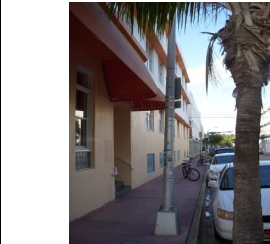
3 Exterior photo looking down city sidewalk
