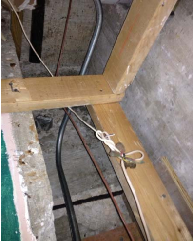
22 Closet photo / reinforced concrete walls & ceiling
