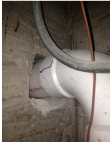
23 Conduit through reinforced concrete in stairway closet
