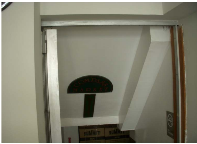
13 Stairway to 7-11 space showing structural beam
