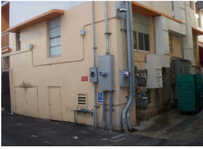
9 SW Corner of building / alley
