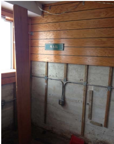
26 Reinforced concrete walls surrounding inaccessible space
