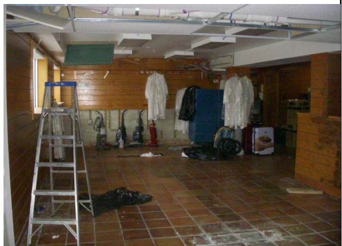
25 Interior photo of west wall of inaccessible space
