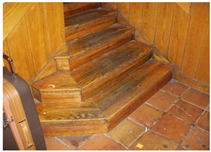
17 Bottom of stairway leading up to exit
