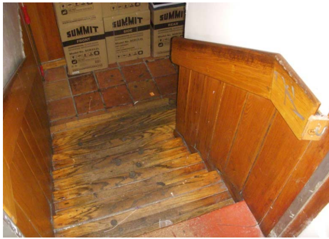
15 Stairway down to proposed 7-11 space
