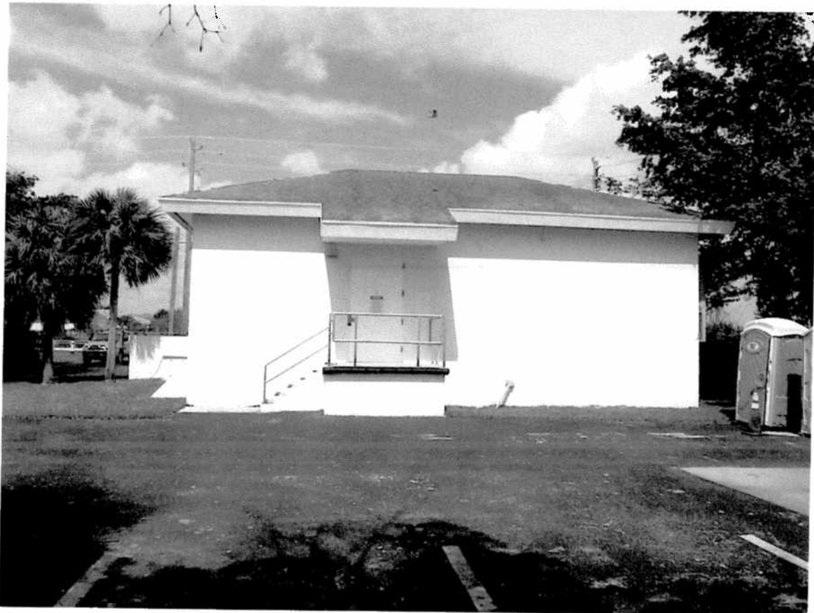
BACK SIDE OF BUILDING (SOUTH FACE)
