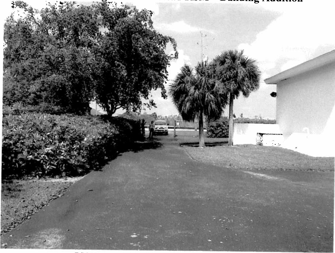
RIGHT SIDE OF BUILDING FACING STREET
