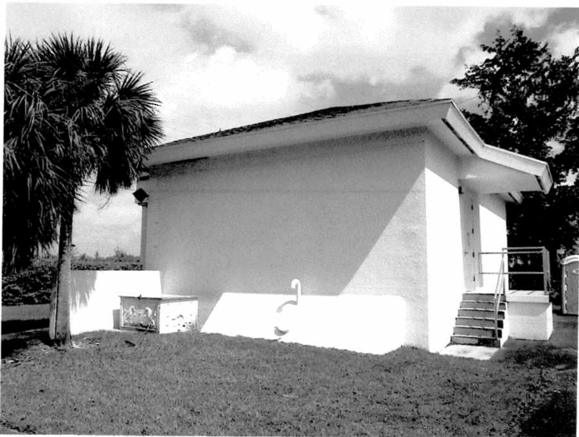
RIGHT SIDE OF BUILDING (WEST FACE)
