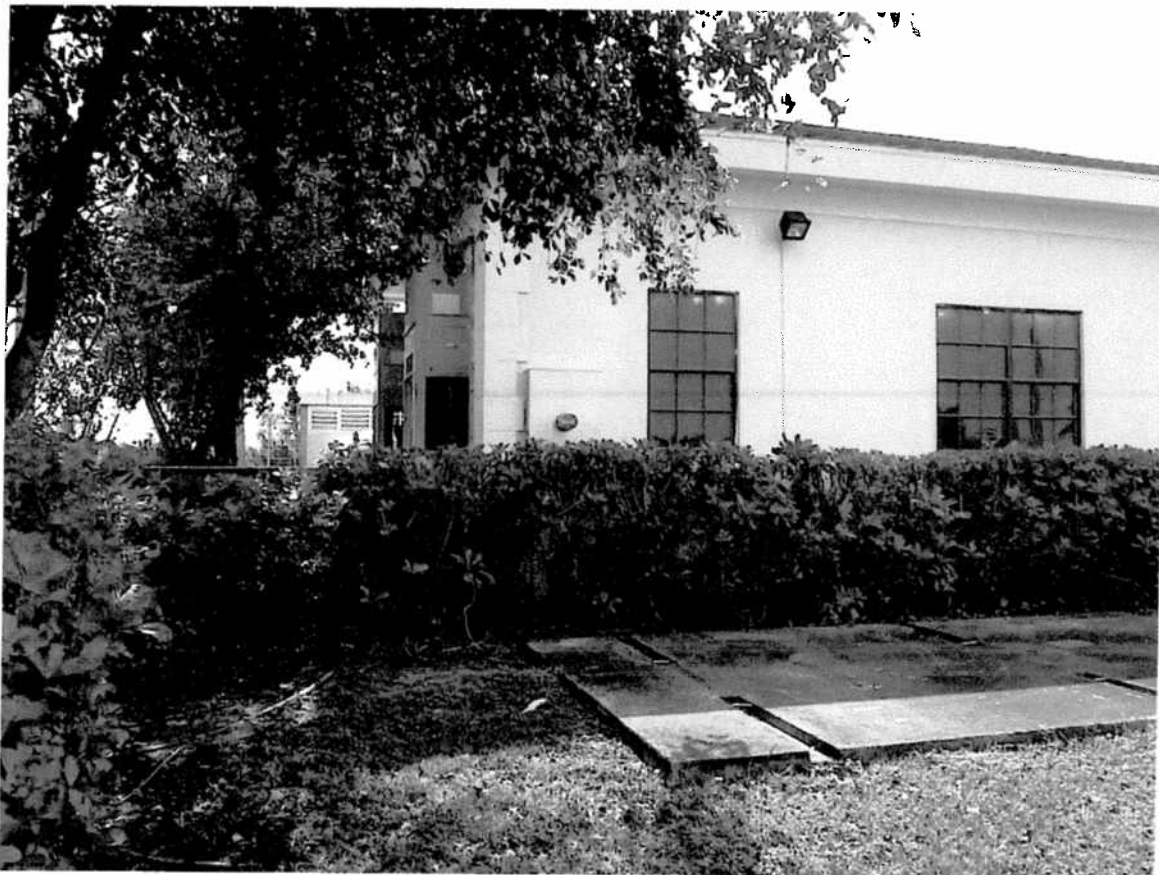
LEFT SIDE OF BUILDING (EAST FACE)
