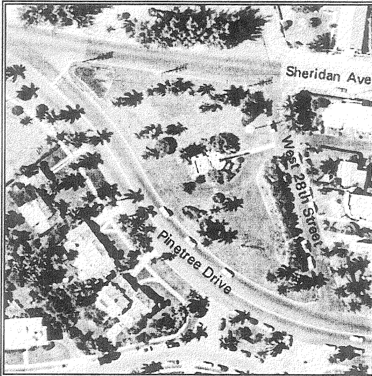
Figure 24 A small addition was built in 1948 on the south side (left) of the 28th Street Obelisk and Pumping Station to house an electrical generator, as seen in this 1954 aerial photo. The original landscape wall and steps may have been removed at the same time this addition was constructed.
