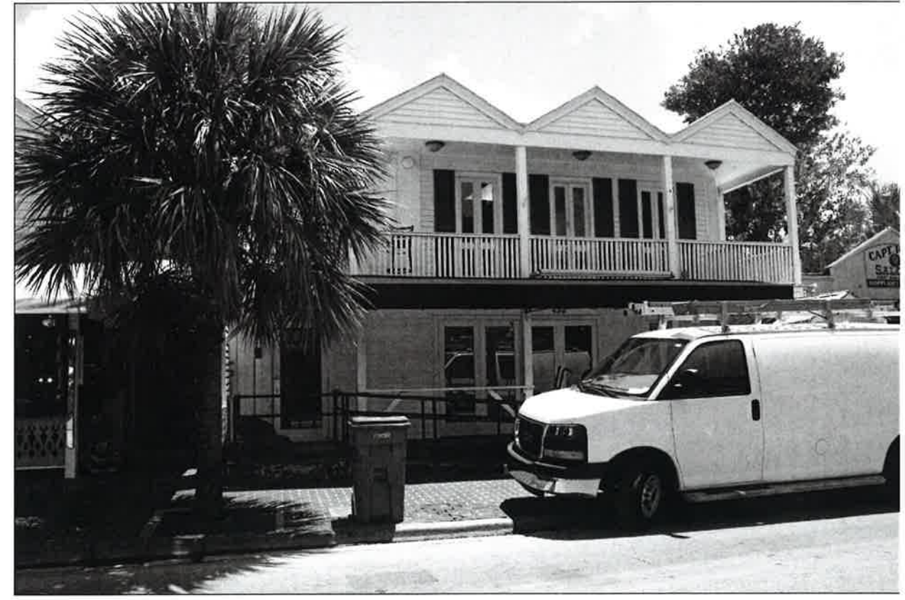
1 PHOTO DETAIL 1 - 430 GREENE STREET (CURRENT) A2
