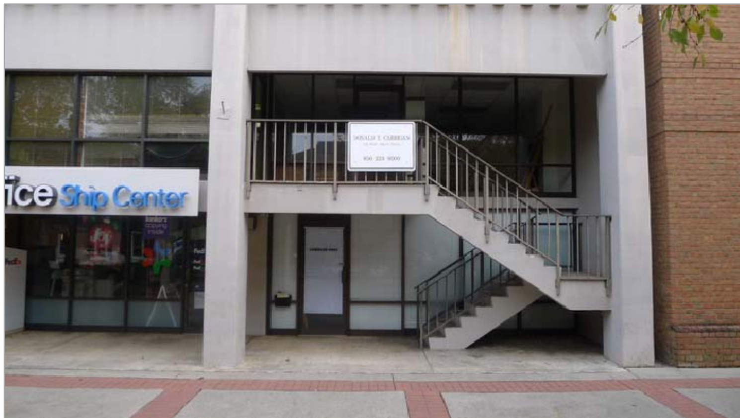
VIEW LOOKING EAST ALONG ADAMS ST.
