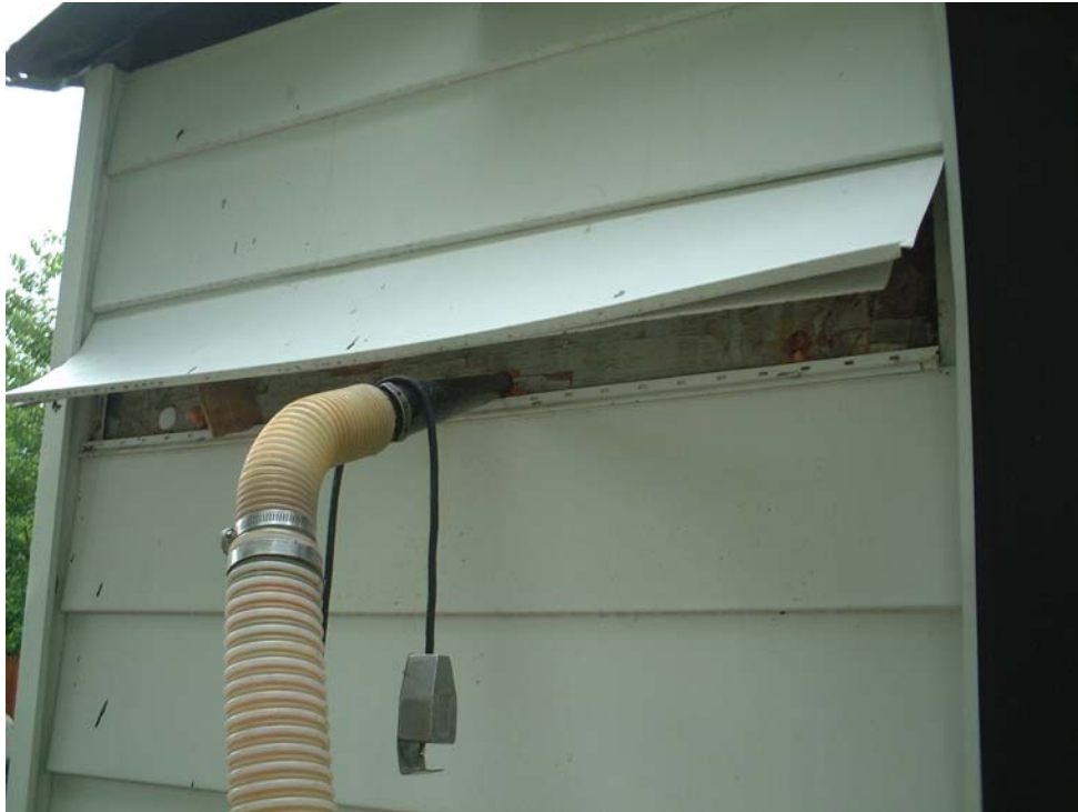
Installation of Blown-in Insulation
