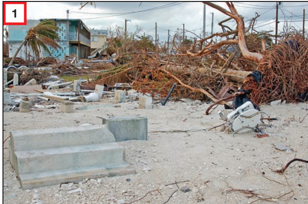
House near shoreline and subject to wave action/ high water velocity was washed off its foundation and destroyed.
