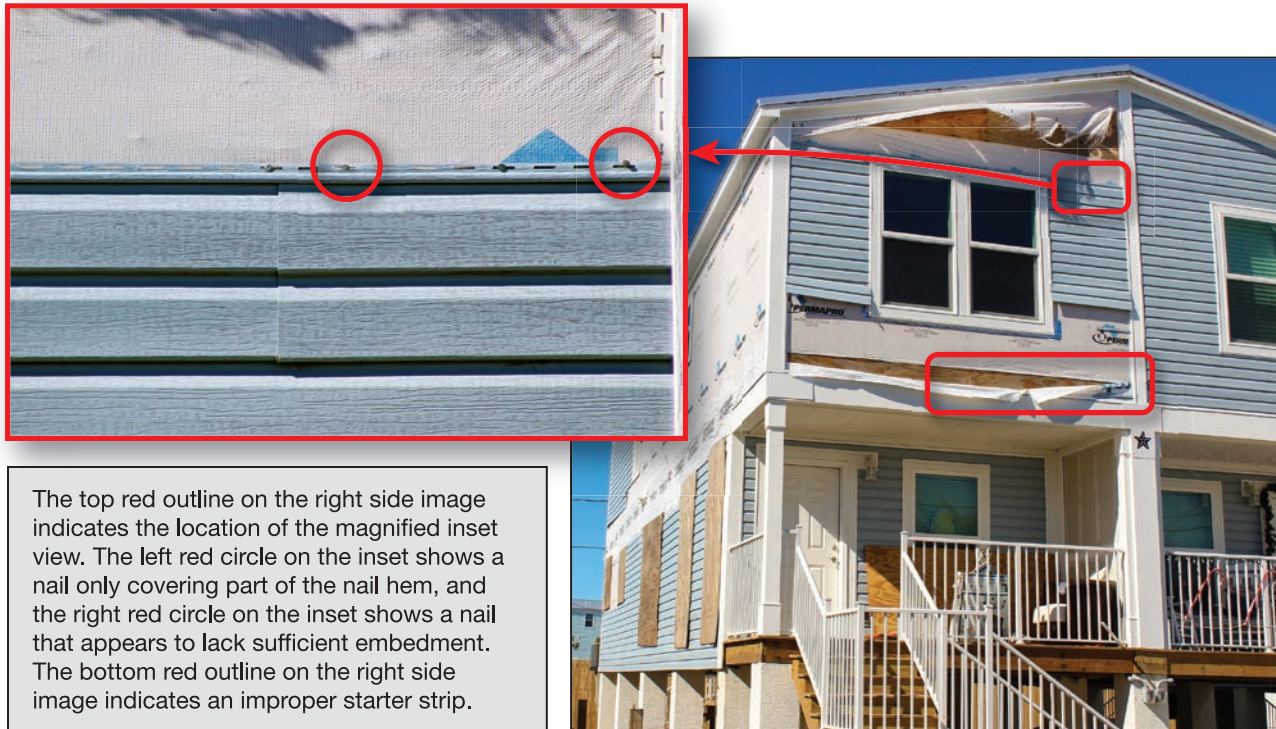
Figure 4-28: Duplex where vinyl siding above the front porch did not comply with manufacturer's installation instructions (EWS = 120 mph; EDWS = 180 mph) (Marathon Key)
