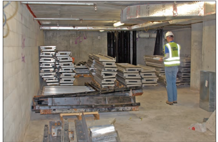
Figure 5: Enclosed storage space for multiple flood panels, stanchions, and hardware
