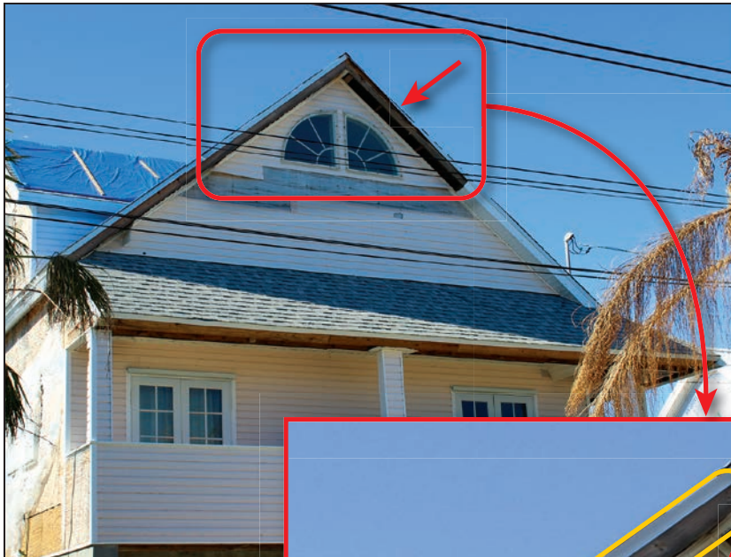
Figure 4-18: House that lost its soffit along the right side of the front-facing gable (EWS = 114 mph; EDWS = 180 mph) (Little Torch Key)
