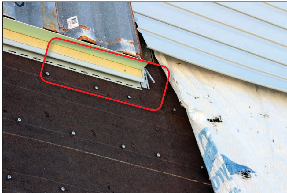
Figure 4-28: Duplex where vinyl siding above the front porch did not comply with manufacturer's installation instructions (EWS = 120 mph; EDWS = 180 mph) (Marathon Key)
