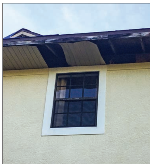
Missing metal soffit panels are shown below damaged fascia; located on the other side of the corner shown in left image.
