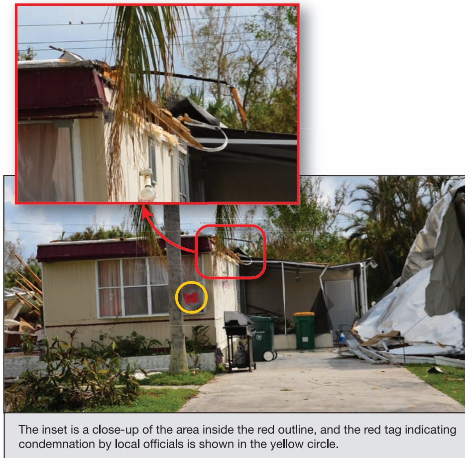
Figure 4-46: MH unit where carport detached from the unit, opening the building envelope across the top of a wall (EWS = 105 mph; EDWS = 166 mph) (Collier County)
