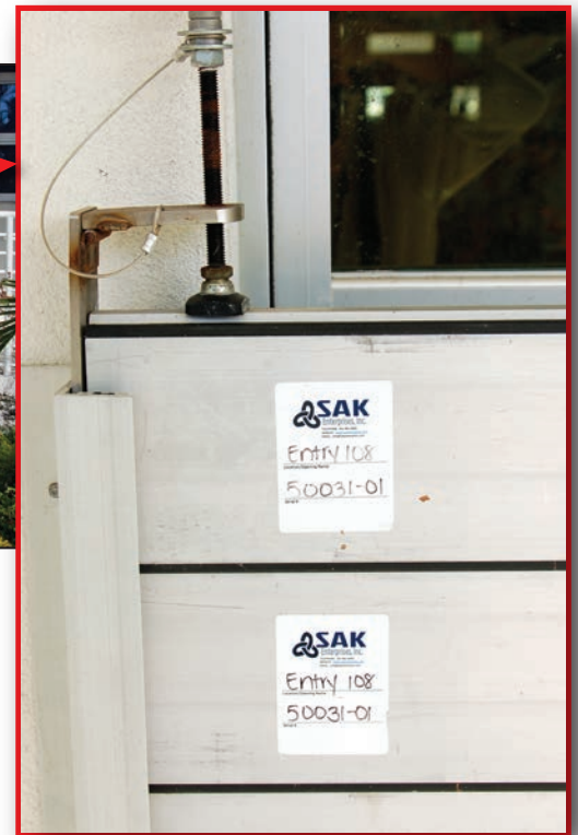
Figure 6: Installed flood panels. Each flood panel has a unique ID number. Also note the tightener bracket at top.
