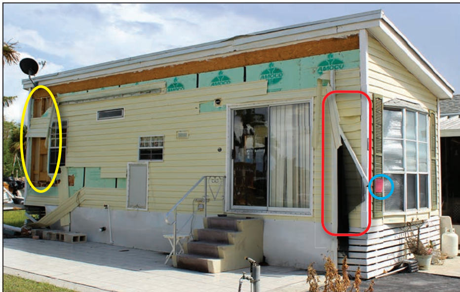
A remnant of the porch is shown in the red outline, and the red tag indicating condemnation by local officials is shown in the blue circle. The yellow oval shows missing sheathing and insulation characteristic of interior walls.
