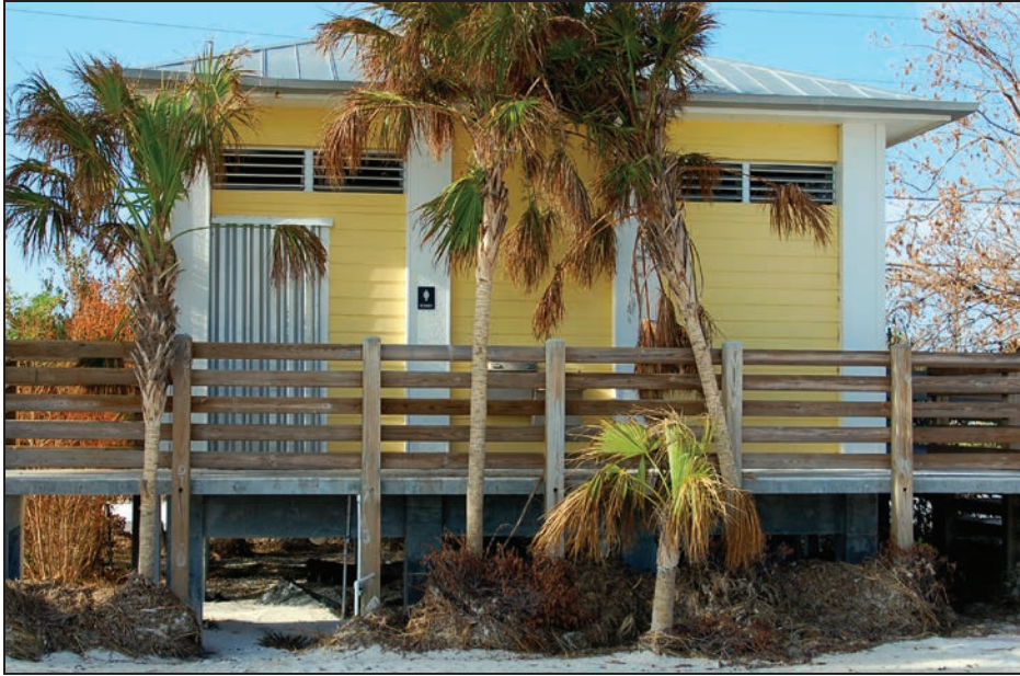
Figure 3-39: Elevated restrooms at Sombra Beach Park without ground-level enclosure and that sustained no flood damage during Hurricane Irma (Site 7; Marathon)
