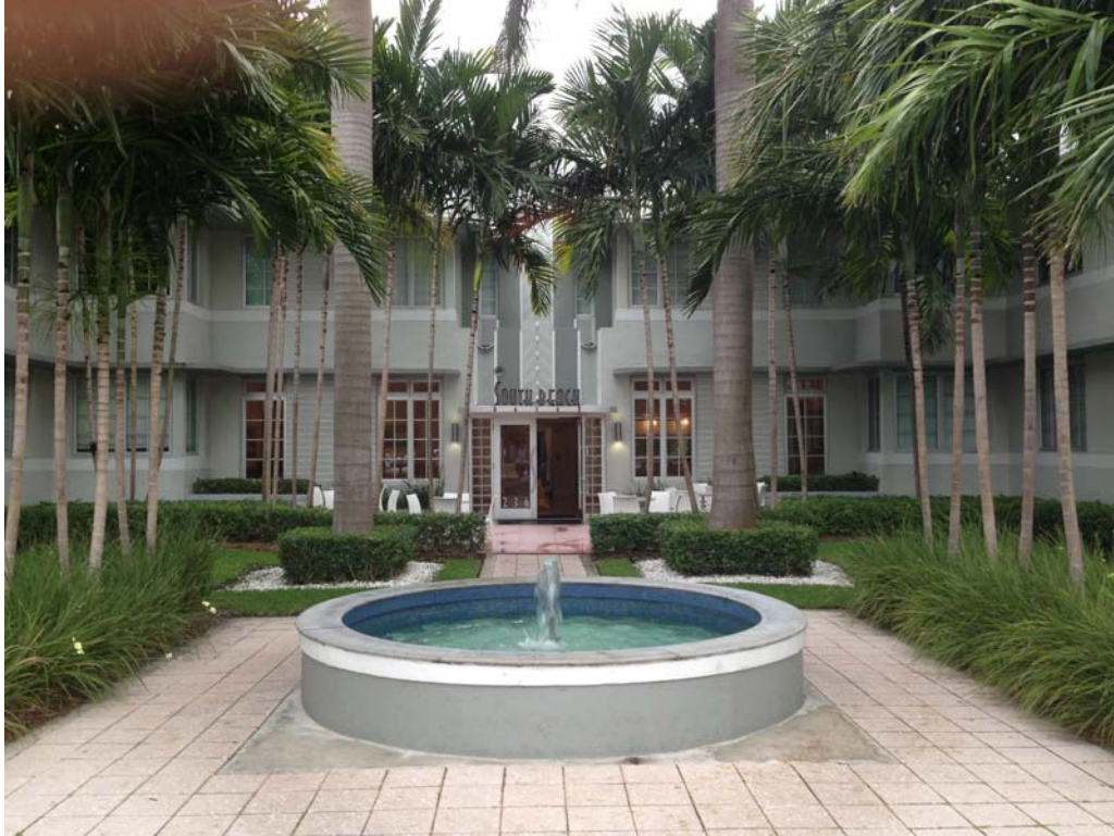
SoBe Hotel: No Level changes from Courtyard to Hotel Lobby
